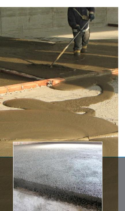
**iSCREE 24** are synthetic polypropylene fibres specifically designed for screeds reinforcements:
