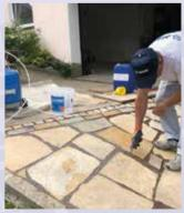
Fill the grouts with 3/6 mm coarse stone chippings and **Mapstone Joint**
