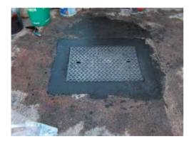
Hi-flow, compensated-shrinkage, rapid-setting and hardening mortar available in grey and back for repairing concrete floors and anchoring manholes, drain covers and street furniture and features.
