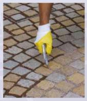
Fill the grout lines with **Mapestone Joint**
