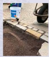
Prepare and apply the mix made up of 3/6 mm coarse stone chippings and **Mapestone Joint**
