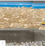
Protective coat of **Mapewash Protex** on all the substrates in and around the floor that could get dirty during the various work phases.
