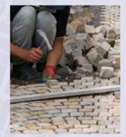
Install the stone blocks on a bed of 4/8 mm or 3/6 mm coarse stone chippings
