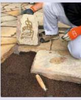
Apply **Mapestone Joint** on the back of the slabs
