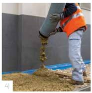
Pouring Mapei Color Paving architectural concrete.
