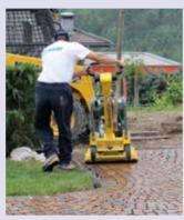
After wetting the surface, use a vibrating plate compactor
