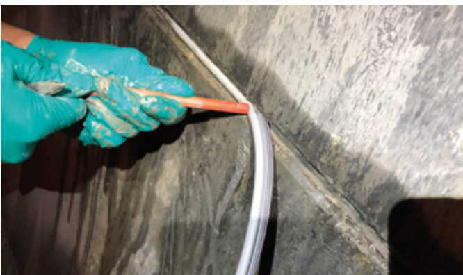
MAPEPLAN JOINT installation by using hand tool
