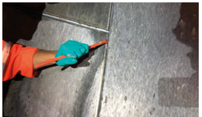
Surface joint cleaning
