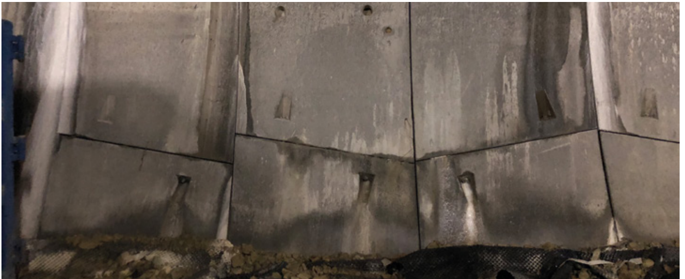
Surface inspection: address the segment joint that shall be sealed
