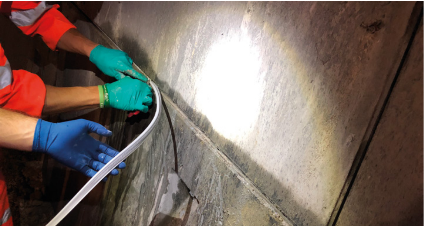
MAPEPLAN JOINT installation
