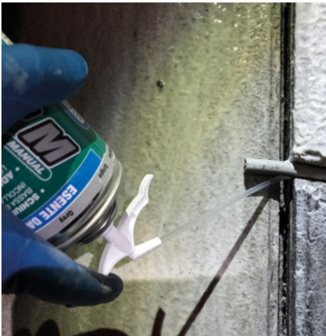
Head joint sealing by using MAPEPUR UNIVERSAL
