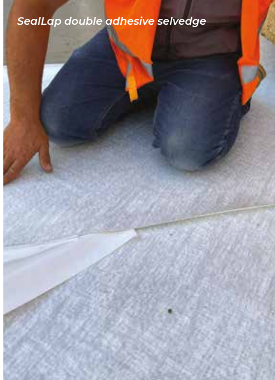
Joining corners of Mapeproof FBH
