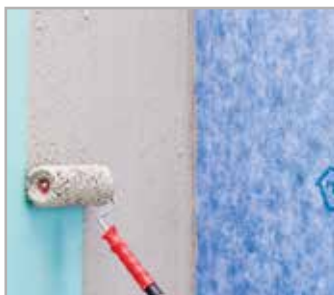
Spreading MAPEGUARD WP ADHESIVE with a roller
