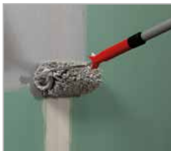
Spreading the first coat of MAPEGUM WPS
