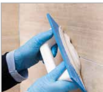
Grouting with FLEXCOLOR 4 LVT
