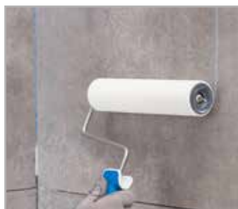
Application of MAPECOAT 4 LVT
