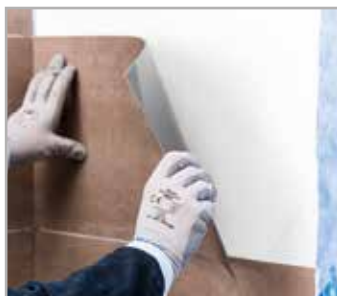
Installation of LVT on wall with ULTRABOND ECO MS 4 LVT WALL&FLOOR
