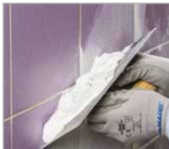
Wall and floor smoothing with PLANIPREP 4 LVT
