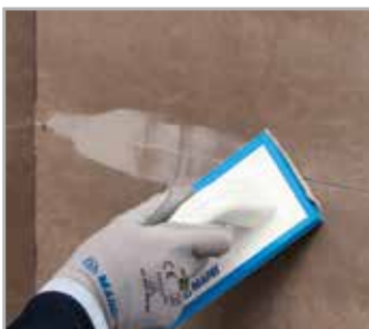
Grouting with FLEXCOLOR 4 LVT
