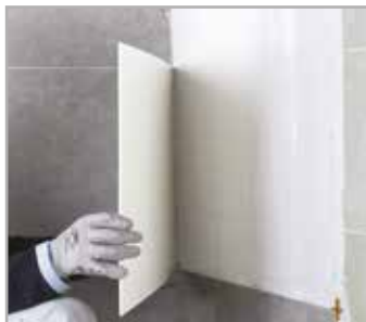
Installation of LVT/SPC with ULTRABOND ECO MS 4 LVT WALL&FLOOR
