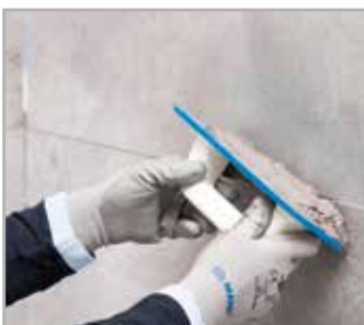
Grouting with FLEXCOLOR 4 LVT
