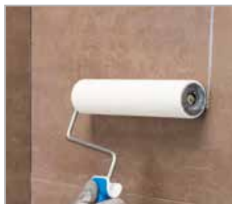
Application of MAPECOAT 4 LVT
