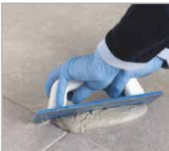
Grouting with FLEXCOLOR 4 LVT
