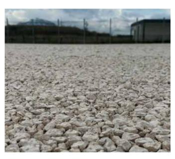
The **Coldpav** system by MAPEI is used to create decorative paving by stabilising soil (either naturally occurring on site or brought in to site) of surface cycle tracks, footpaths and dirt tracks.
