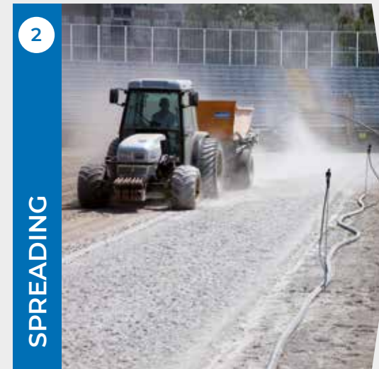
2 SPREADING Spreading on the Mapesoil 100 with a sandblaster
