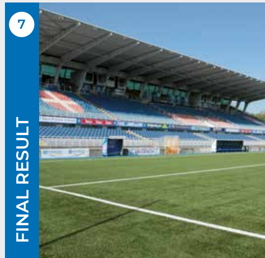
7 FINAL RESULT Synthetic grass playing field with horizontal drainage made using Mapesoil 100
