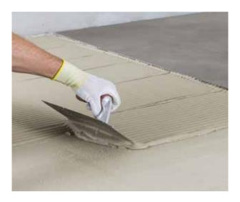
One-component, high-performance, grey and white deformable, lightweight, cementitious adhesive with no vertical slip, extended open time, and extremely high yield. It is easy to apply by trowel and features excellent wetting capacities, Low Dust technology, very low emission of volatile organic compounds and fully offset Greenhouse Gas Emissions. It is classified as C2TES1 according to the standards EN 12004 and ISO 13007-1, as well as EMICODE EC1 Plus by the GEV.
