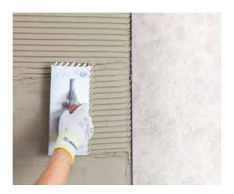
One-component, rapid-setting and -hydration, high-performance, highly deformable, grey and white lightweight, cementitious adhesive with extended open time, and extremely high yield. It is easy to apply by trowel and features excellent wetting capacities, Low Dust technology, and very low emission of volatile organic compounds. It is classified as C2FES2 according to the standards EN 12004 and ISO 13007-1, as well as EMICODE EC1 Plus by the GEV.
