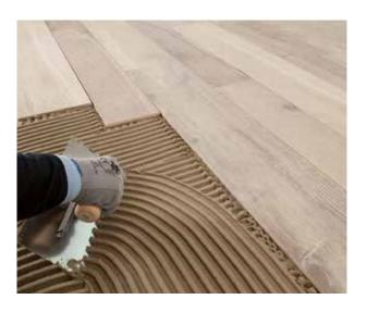
**One-component**, high-performance, moderately deformable, grey and white **lightweight**, cementitious adhesive with no vertical slip, extended open time, and high yield. It is easy to apply by trowel and features excellent wetting capacities, Low Dust technology, and very low emission of volatile organic compounds. It is classified as C2TE according to the standards EN 12004 and ISO 13007-1, as well as EMICODE EC1 Plus by the GEV.
