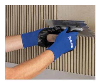
**One-component**, high-performance, **highly deformable**, grey and white **lightweight**, cementitious adhesive with extended open time, and extremely high yield. It is easy to apply by trowel and features excellent wetting capacities, Low Dust technology, and very low emission of volatile organic compounds. It is classified as C2ES2 according to the standards EN 12004 and ISO 13007-1, as well as EMICODE EC1 Plus by the GEV.
