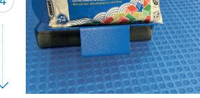
Go over the membrane with **Mapeguard Roller** and press it down (maximum 35 kg).
