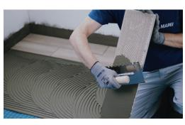
Install ceramic or stone tiles with a suitable **Mapei** adhesive of at least C2 class.
