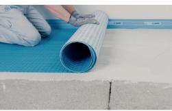
Lay **Mapeguard UM 35** membrane over the adhesive while it is still wet.
