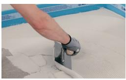
Spread the adhesive over the surface of the substrate with a 5 notches trowel.
