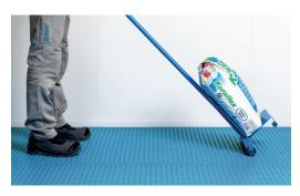
Go over the membrane with **Mapeguard Roller** and press it down (maximum 35 kg).
