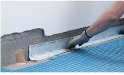
Perimetrally waterproof with **Mapeband Easy**, bonded with **Mapeguard WP Adhesive** (3 mm notches trowel).
