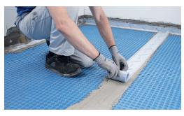
Waterproof joints between adjacent sheets with Mapeband Easy, bonded with Mapeguard WP Adhesive (3 mm notches trowel).
