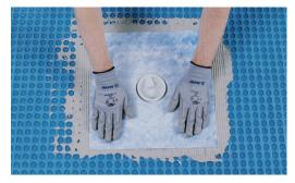
Waterproof drains with **Drain Vertical/Drain Lateral.**
