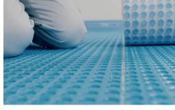
Apply **Mapeguard UM 35** rolls leaving a 3-5 mm gap between the sheets.
