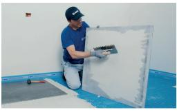
Install ceramic or stone tiles with a **Mapei** suitable adhesive of at least C2 class.
