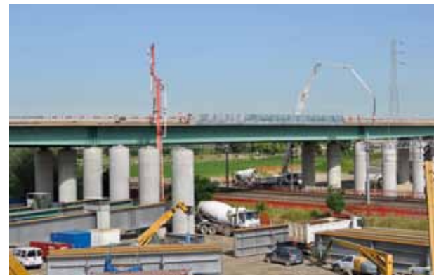
Slab on viaduct
