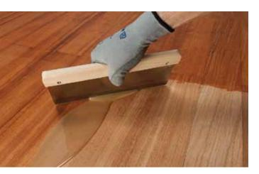
Water and oil-repellent oil/wax finish with very little odour used to protect wooden surfaces and give them a delicate, warm colour.
