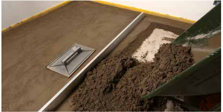
Installing a screed made from TOPCEM PRONTO
