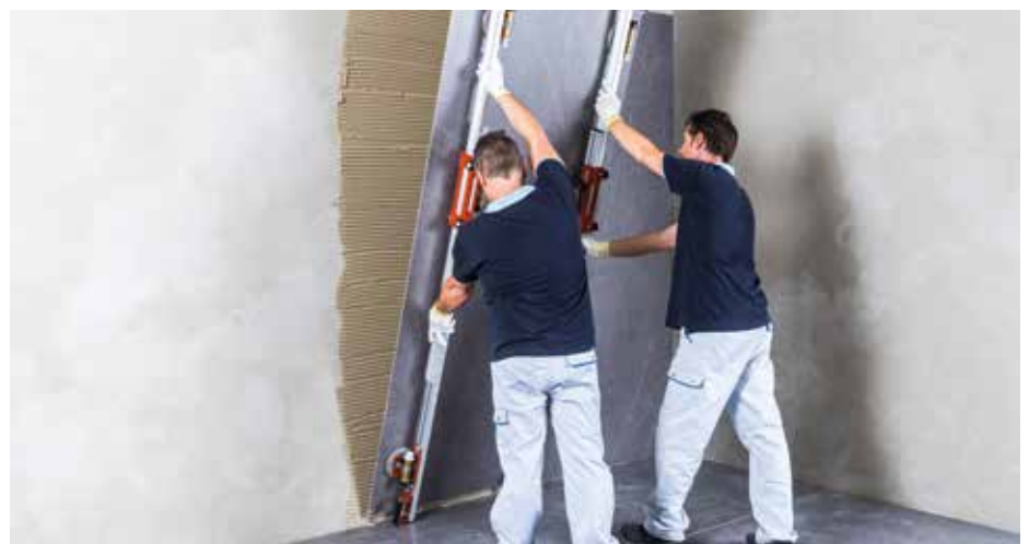
Installing a wall tile
