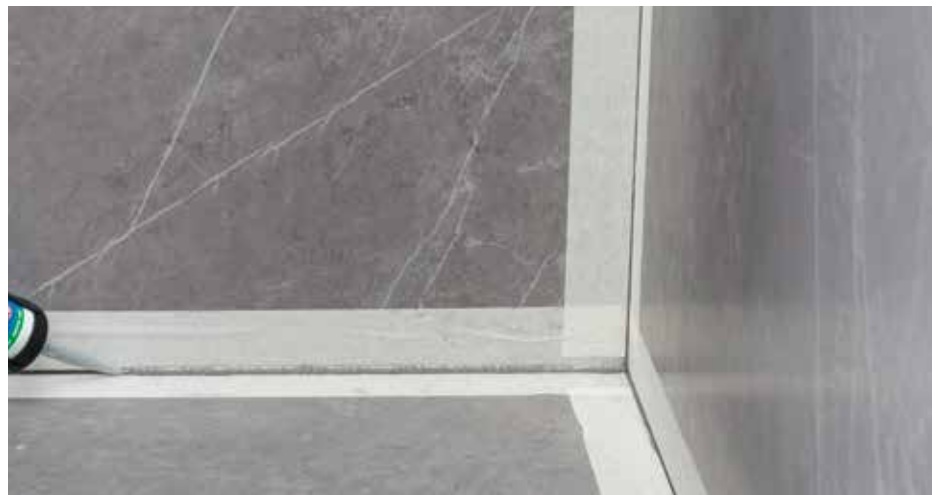
Perimeter joint sealed with MAPESIL AC
