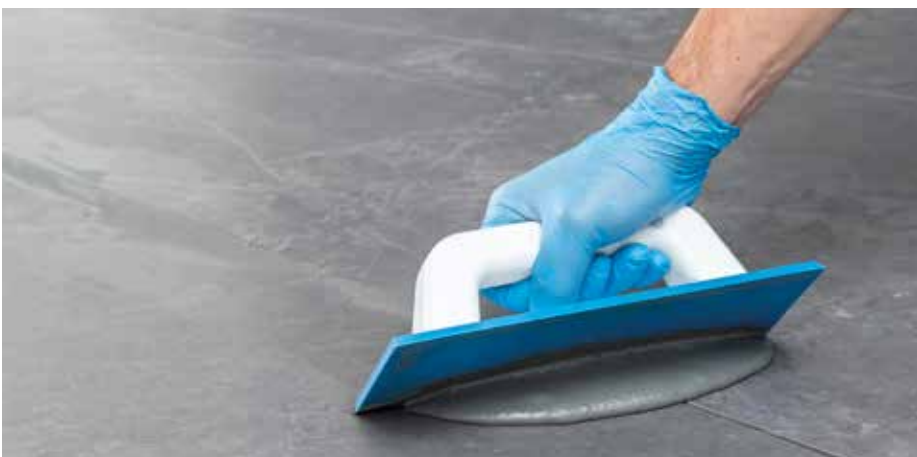
Grouting the tiles
