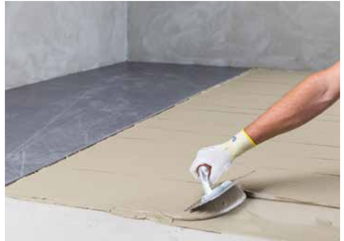
The adhesive is spread in the same direction on the back of the tile and on the substrate
