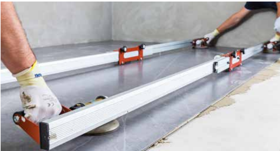
Installing a tile
