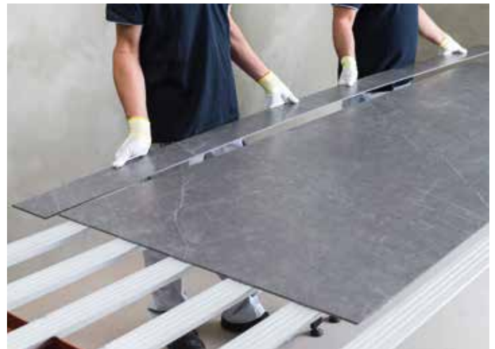
Breaking the tile in two
