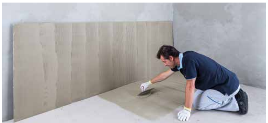
Installing a tile using the double-buttering technique
