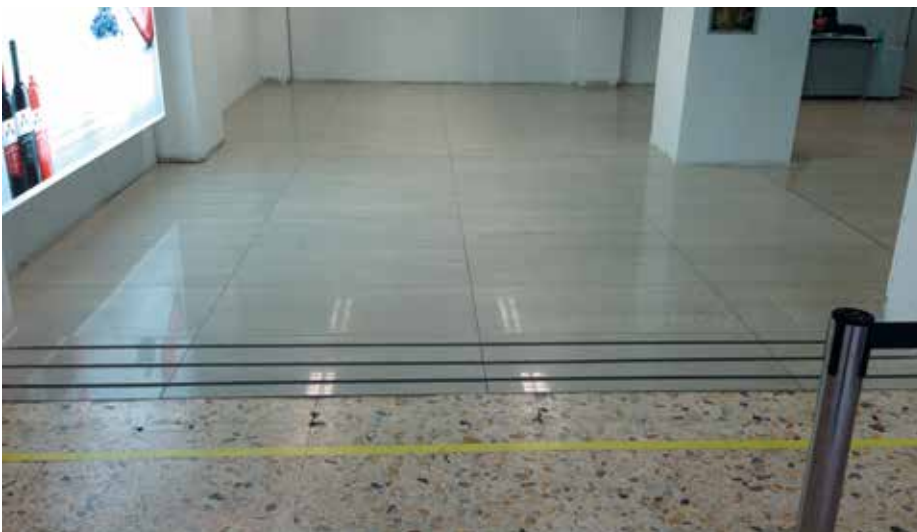
Installing tiles over an old floor
