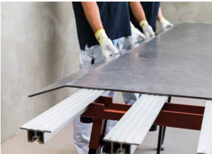
Breaking the tile in two
