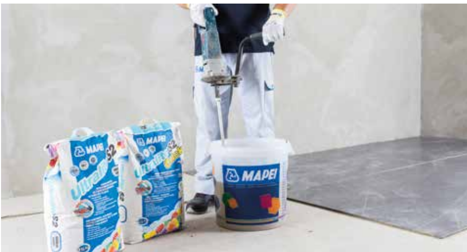
Mixing the adhesive
