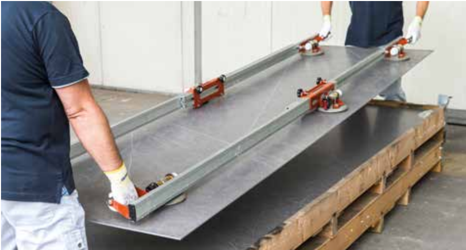
Correct handling of a tile
