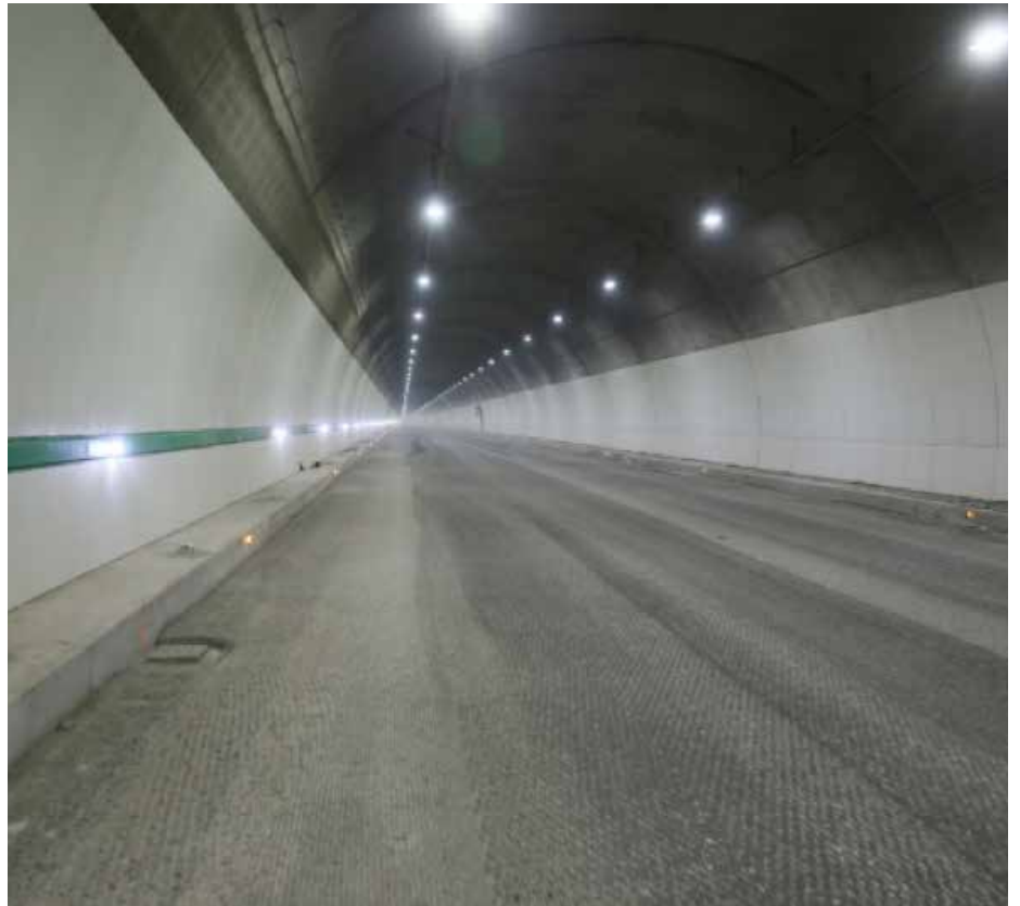
ROAD TUNNEL IN THE VALICO BY-PASS, CASTIGLIONE DE' PEPOLI (BO) - ITALY
