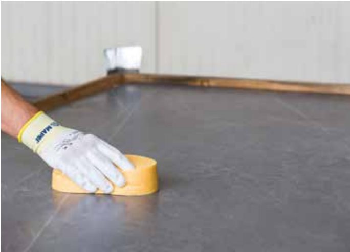
Cleaning the surface of the tile and suction cup
