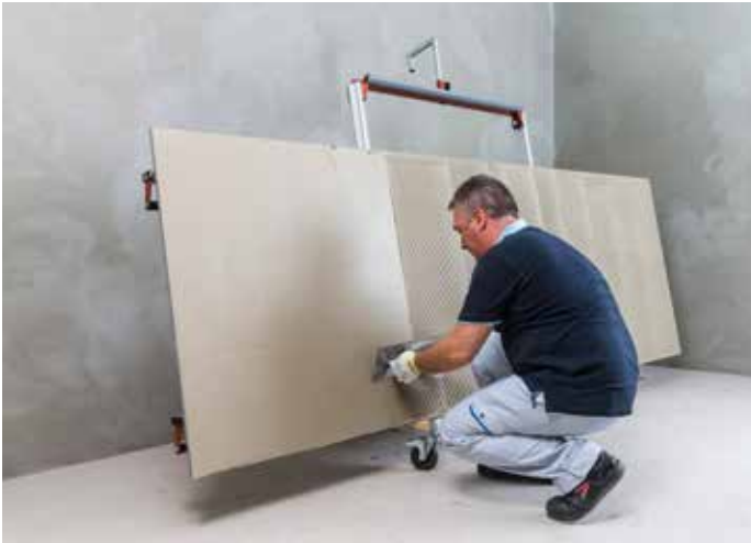
The adhesive is spread in the same direction on the back of the tile and on the substrate
