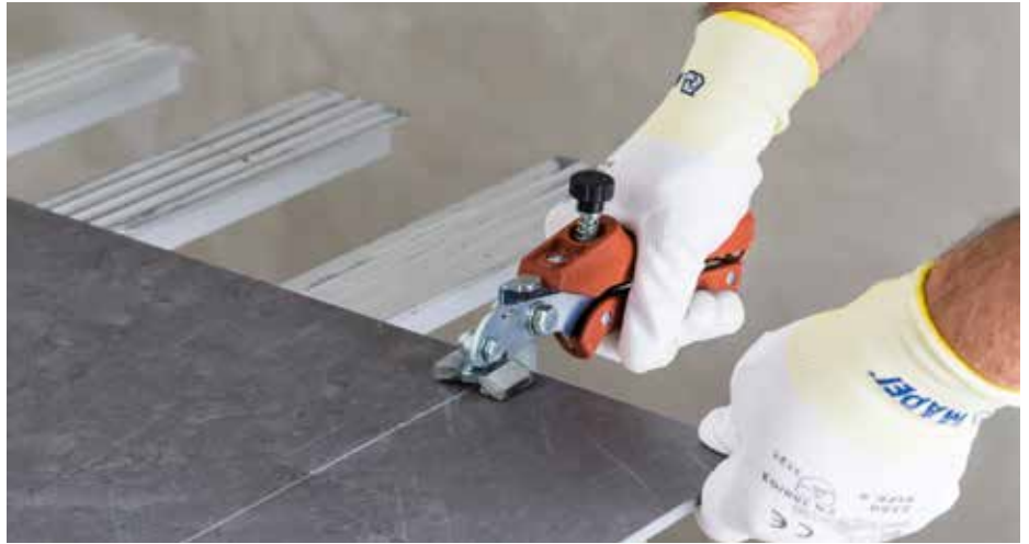
Creating a fracture with tile snips
