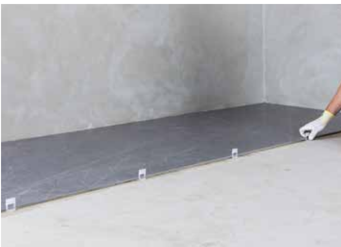
Placing the spacers in position
