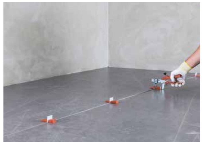
Placing the spacers in position
