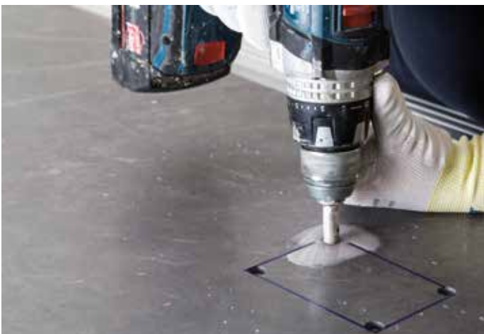
Sequence to make a rectangular hole
