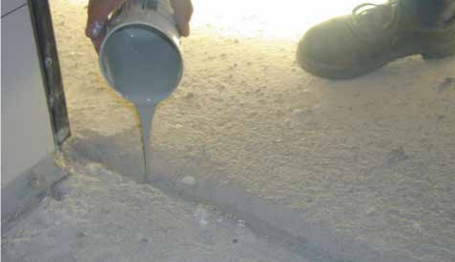
Sealing cracks in a substrate with EPORIP
