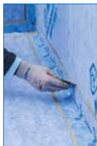
Application of Mapeguard ST
