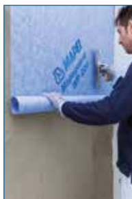
Application of Mapeguard WP 200
