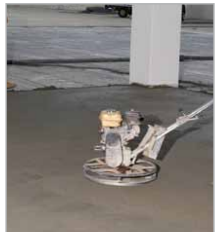
Fig. 7.7 - Finishing the surface of a screed with a power float
