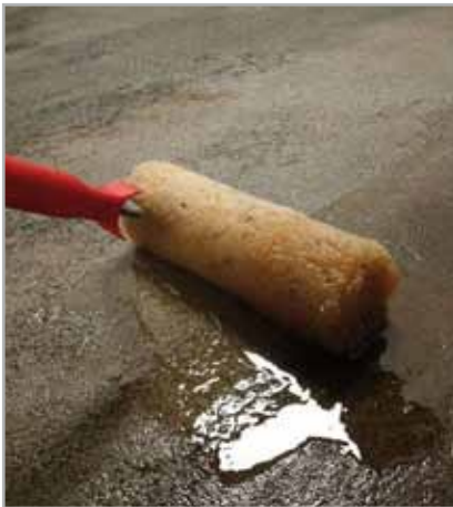
Fig. 8.11 - Applying PRIMER MF on the surface of a screed
