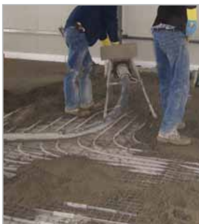
Fig. 4.7 - Laying a screed with embedded heated elements for an underfloor heating system.
