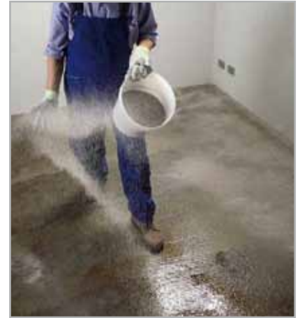
Fig. 8.12 - Dusting the surface of a screed with sand after applying a coat of PRIMER MF
