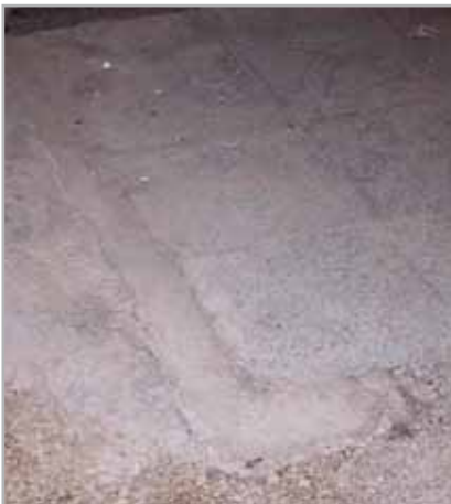
Fig. 7.3 - Sealing a chase in existing flooring by applying bonding slurry on the contact surfaces between the existing and repaired surfaces
