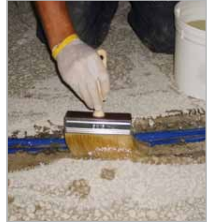
Fig. 8.7 - Applying bonding slurry made from epoxy resin (PRIMER MF)
