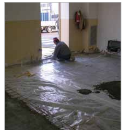
Fig. 4.2 - Laying an unbonded screed on polyethylene sheets
