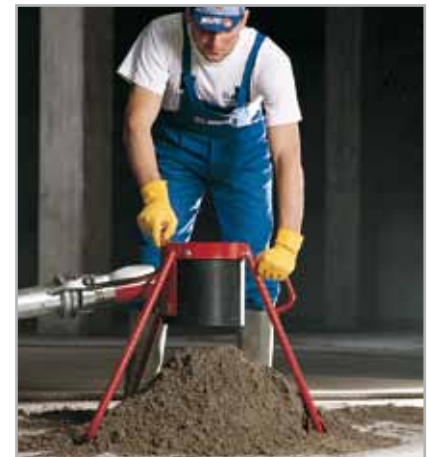
Fig. 6.2 - Batching a TOPCEM/TOPCEM PRONTO mix
