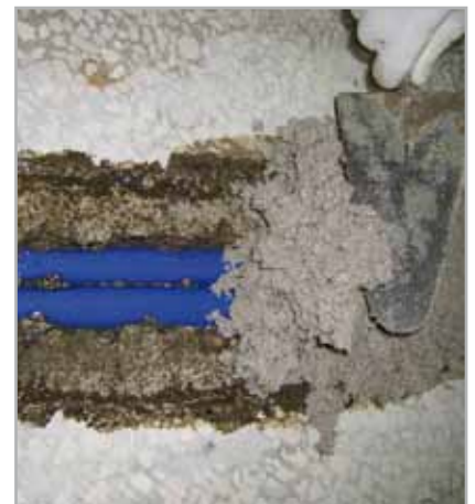
Fig. 8.8 - Filling fractures with MAPEFLOOR EP19
