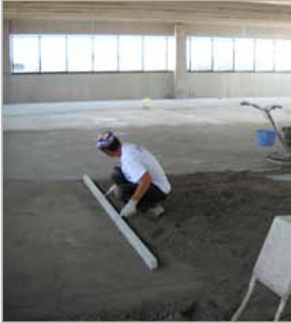
Fig. 6.3 - Levelling off the surface of TOPCEM/TOPCEM PRONTO mix
