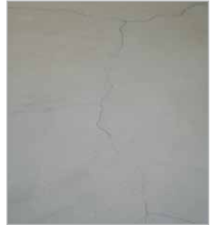
Fig. 8.1 - Cracked screed
