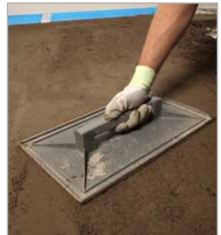
Fig. 7.6 - Float-finishing the surface of a screed
