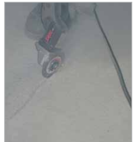
Fig. 8.2 - Opening cracks in a screed with an angle grinder
