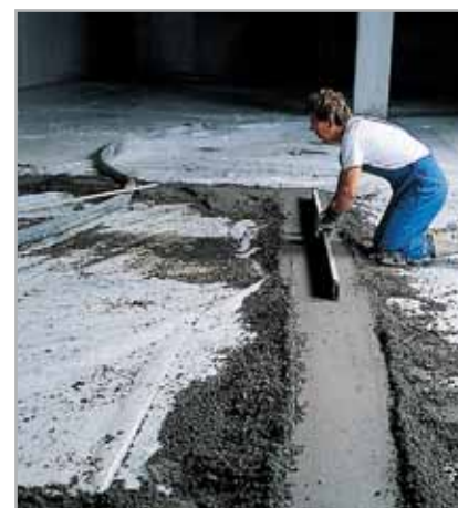
Fig. 7.1 - Forming levelling strips
