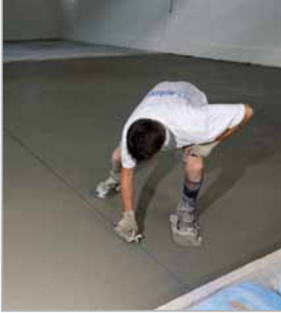
Fig. 7.8 - Forming check joints in a screed
