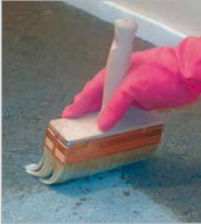
Fig. 8.13 - Brush-applying PRIMER G diluted with water on the surface of a screed
