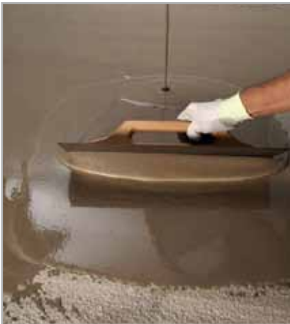
Fig. 8.14 - Creating a flat surface on a screed by applying a layer of ULTRAPLAN
