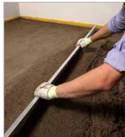
Fig. 3.4 - Using a straight-edge on the screed
