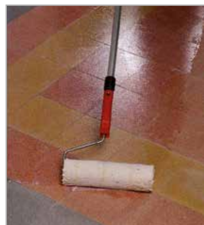
Fig. 3.6 - Applying a primer as bonding promoter
