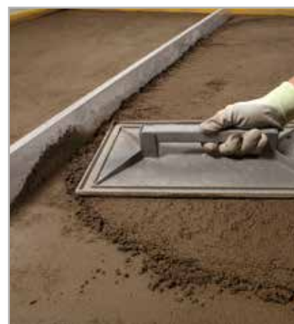
Fig. 3.5 - Floating the screed's surface
