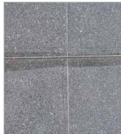
Fig. 4.10 - Example of staining on natural stone installed with acetic cross-linking silicone sealant
