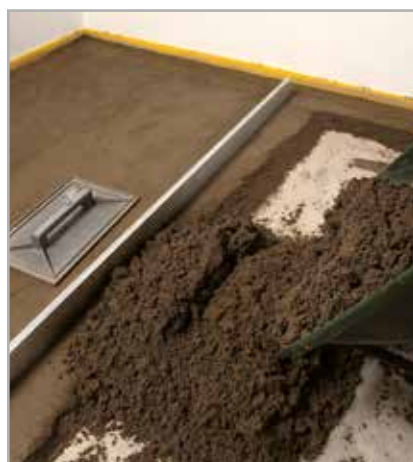
Fig. 3.3 - Carrying out a MAPECEM PRONTO screed
