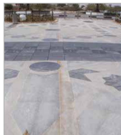
Fig. 4.11 - Example of staining on natural stone installed with acetic cross-linking silicone sealant
