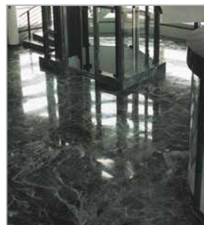
Fig. 4.9 - Example of installation of Verde Alpi marble flooring with KERALASTIC – Rolex Hall – Bienne – Switzerland
