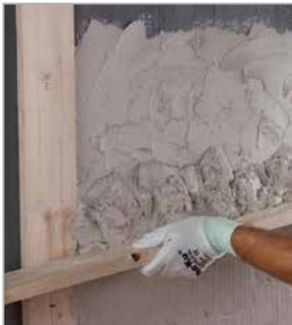
Fig. 3.8 - Evening out a concrete wall with NIVOPLAN+PLANICRETE
