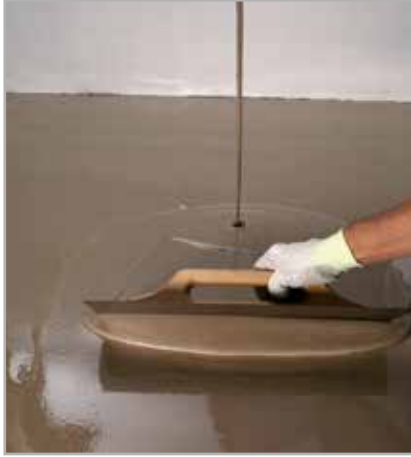
Fig. 3.7 - Levelling a cementitious screed with ULTRAPLAN
