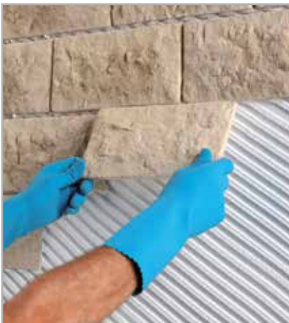
Fig. 5.1 - Laying engineered decorative elements with FIX & GROUT BRICK
