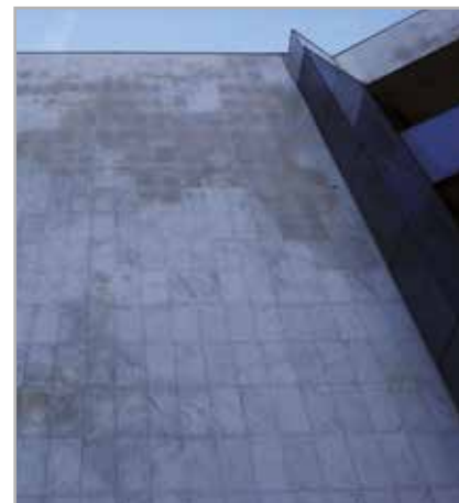
Fig. 2.5 - Example of stains caused by pyrite on white Carrara marble
