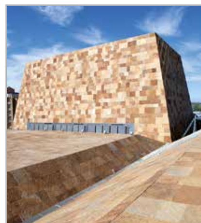
Fig. 4.3 - Example of installation of natural stone on façade - "La Llotja" Congress Centre, Lleida - Spain
