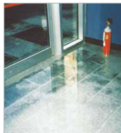
Fig. 2.6 - Example of stains on a granite floor
