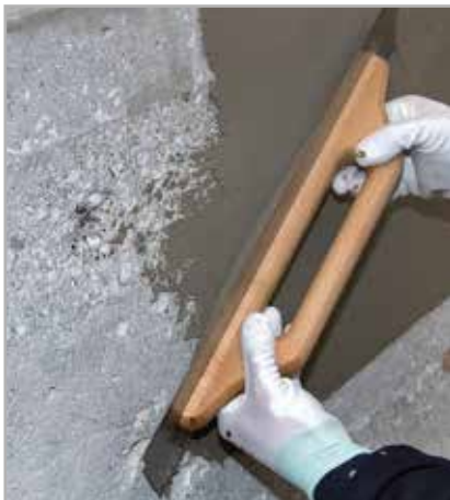
Fig. 3.9 - Evening out a wall with PLANITOP FAST 330
