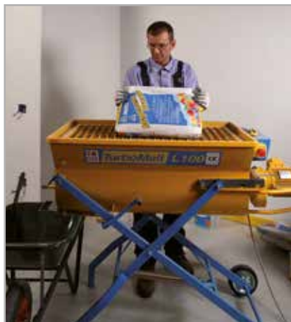
Fig. 3.1 - Mixing MAPECEM PRONTO screed
