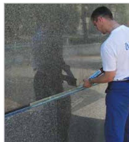
Fig. 4.12 - Sealing joint on façade with MAPESIL LM
