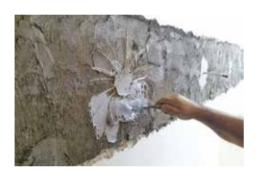
Application of an FRCM system to prevent collapse of dividing and buffer . walls
