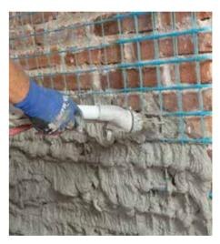
Application of Mapenet EMR 66 system and MapeWall Render & Strengthen, for CRM strengthening of load-bearing masonry
