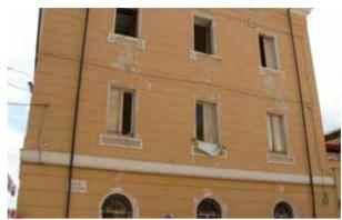
Shear cracks in load-bearing walls
