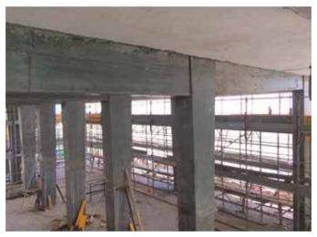
Strengthening of a beam and pillar with a compact jacketing
