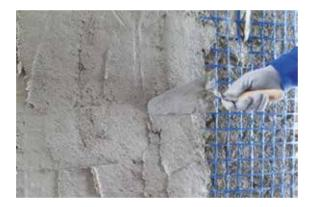
Application of a strengthening package to increase shear-tensile and compressive strength
