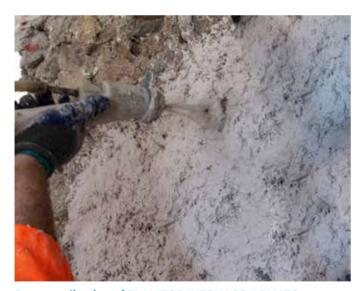
Spray application of PLANITOP INTONACO ARMATO on bearing stone masonry
