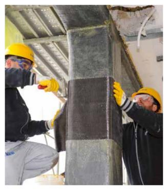
Strengthening of a beam-pillar joint with MAPEWRAP C SYSTEM
