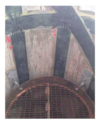
Strengthening of a brickwork chimney with MAPEWRAP C SYSTEM
