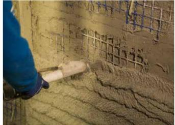
Application of Mapenet EM 40 and MapeWall Render & Strengthen, for CRM strengthening of load-bearing masonry
