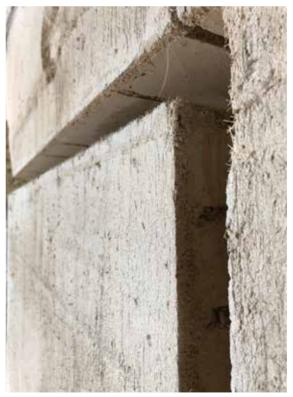
Section for on-site testing of brick masonry reinforced using PLANITOP INTONACO ARMATO
