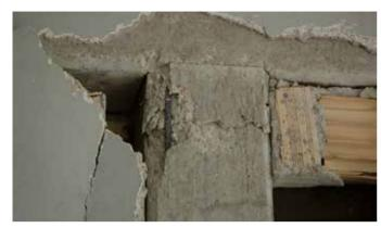
Localised interaction between buffer walls and the reinforced concrete frame
