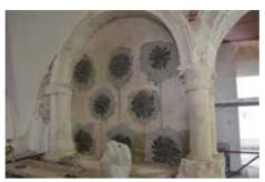
Extra mechanical connection with carbon fibre bows
