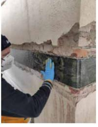
**Binding through** FRP system and creating connections using MapeWrap C Fiocco
