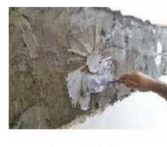
FRCM applied as anti-tipping system connected using MapeWrap SG Fiocco
