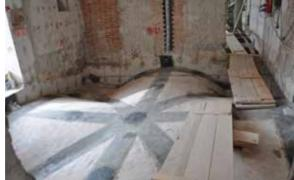
Strengthening for the extrados of vaults through FRP system and creating connections using MapeWrap B Fiocco
