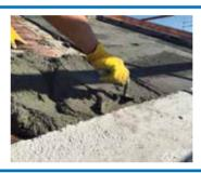
The high fibre content of the product means much less or even no traditional reinforcement is required, as specified in the reference document CNR DT 204/2006; the thickness of the layer of **PLANITOP HPC** applied varies from 20 mm to 40 mm.
