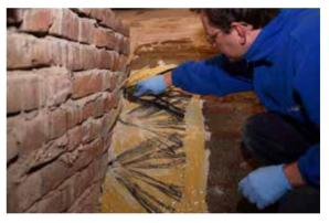
Preparation of connections to vault thrusts using MapeWrap C Fiocco
