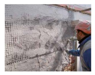
Application of a compact strengthening system to increase the shear-tensile strength of bay walls
