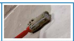
One-component, ready-to-use, polyurethane dispersion-based adhesive with very low emission of volatile organic compounds (VOC) for impregnating MAPEWRAP EQ NET bi-directional, primed glass fibre fabric.
