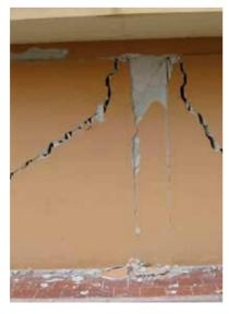
Shear failure of partition walls
