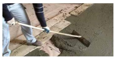
Strengthening of the extrados of a wooden floor
