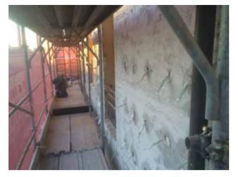
FRCM system connection on masonry using MapeWrap G Fiocco
