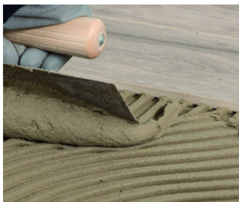
Bonding "imitation wood" effect porcelain floor tiles
