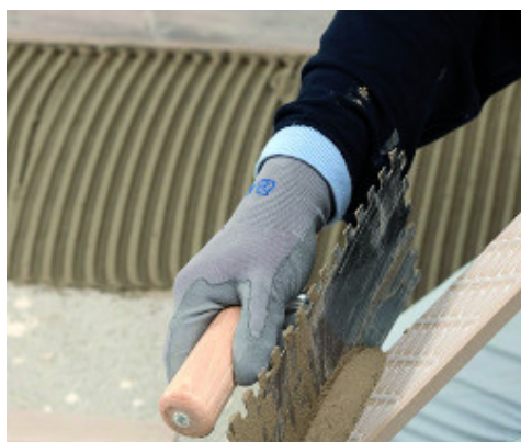
Application with the back-buttering technique
