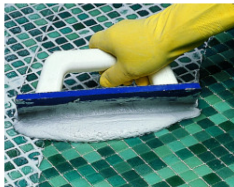
Grouting glass mosaic with Keracolor FF mixed with Fugolastic
