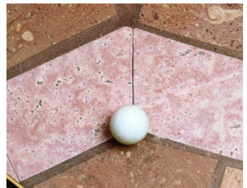
Terracotta floor polished in situ, grouted with Keracolor GG mixed with Fugolastic
