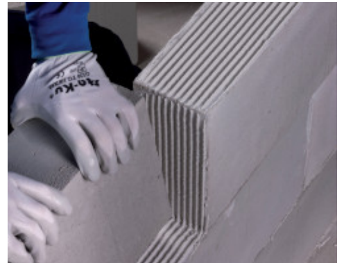
Laying blocks on Porocol FF still fresh
