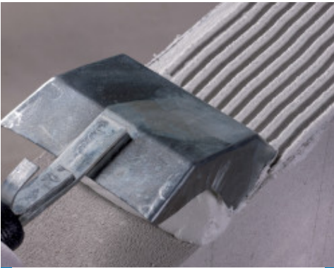
Laying Porocol FF on the surface of the wall with a special notched trowel
