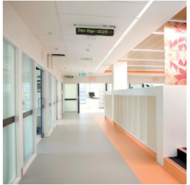
An example of an installation of linoleum on a surface levelled with Ultraplán - Victorian Comprehensive Cancer Centre - Melbourne - Australia
