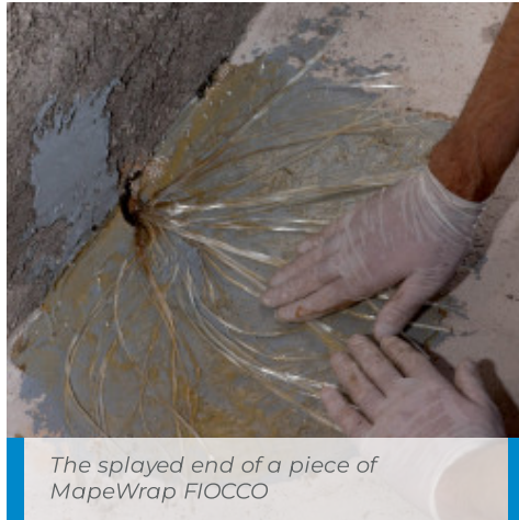
Impregnating a portion of MapeWrap FIOCCO
