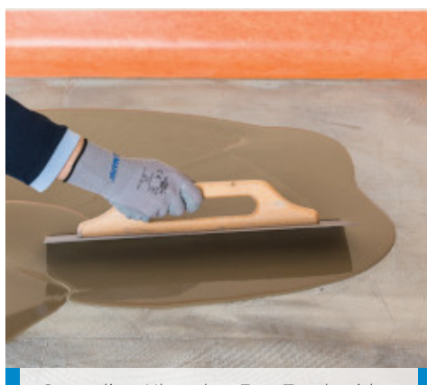
Spreading Ultraplan Fast Track with a metal trowel
