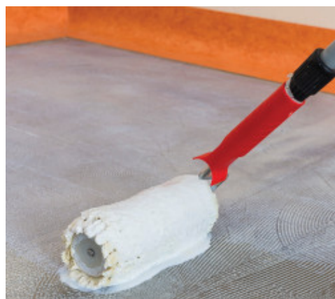
Application of Eco Prim T with a roller
