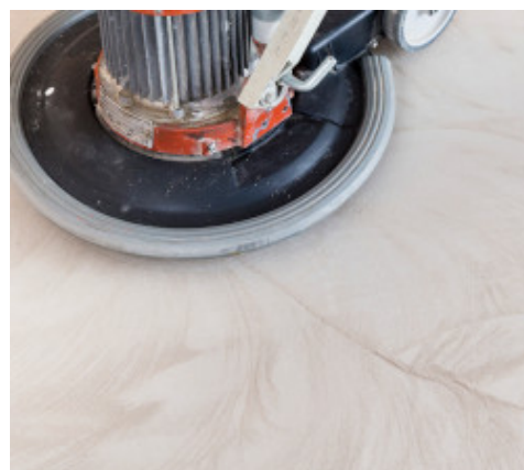
Grinding after 2 hours
