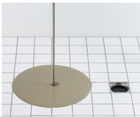
Application of Planex HR on existing ceramic in damp surroundings
