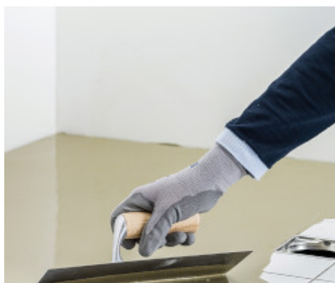
Application of Planex HR with a metal trowel
