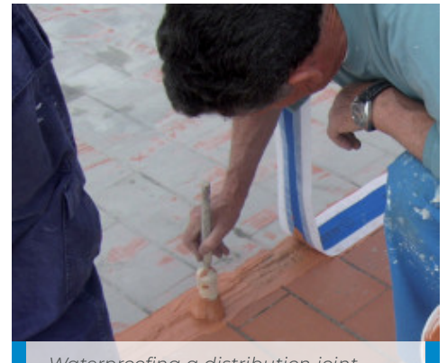
Waterproofing a distribution joint with Mapeband fixed in place with Aquaflex Roof
