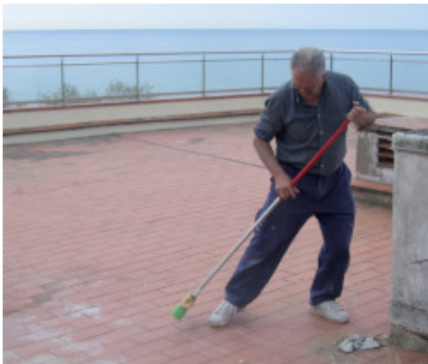
Cleaning a substrate before applying Aquaflex Roof
