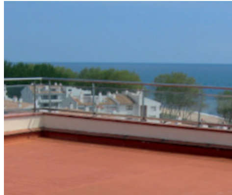
Paving slab waterproofed with Aquaflex Roof
