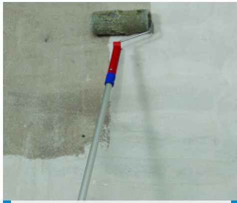
Application of the first layer of MAPEWRAP EQ ADHESIVE
