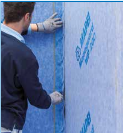
Application of MAPEGUARD ST onto MAPEGUARD WP ADHESIVE
