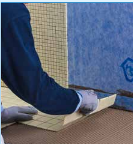
Tile installation with a cementitious tile adhesive
