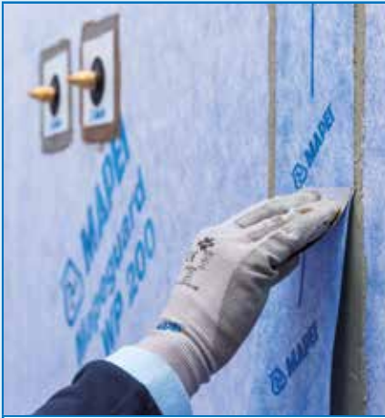
Application of MAPEGUARD ST
