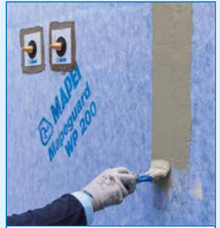
Application of MAPEGUARD WP ADHESIVE before MAPEGUARD ST to seal the junctions between two adjoining sheets
