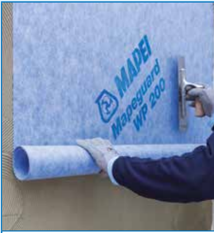
Laying the first sheet of MAPEGUARD WP 200
