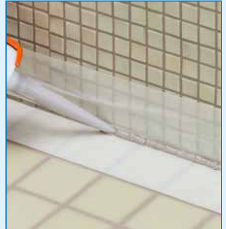
Application of the sealant in all corners
