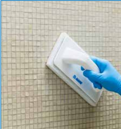
Cleaning off the glass mosaic with a damp Scotch-Brite® pad
