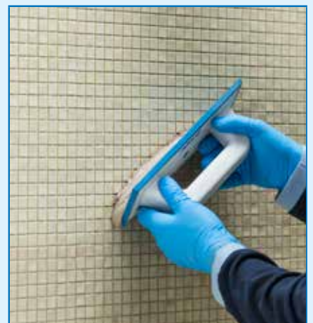
Grouting of the joints
