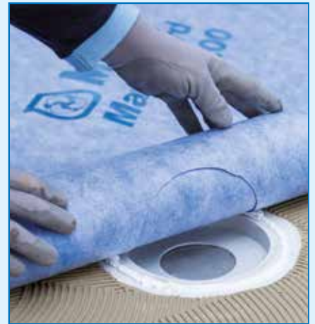
Laying of MAPEGUARD WP 200
