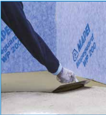
Application of the cementitious tile adhesive
