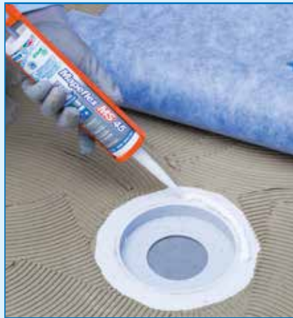
Application of MAPEFLEX MS 45 around the drain
