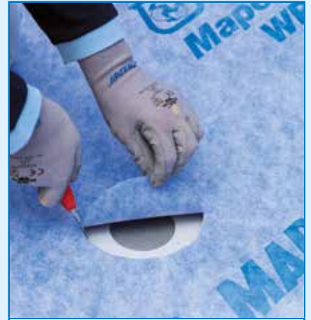
Cutting the membrane
