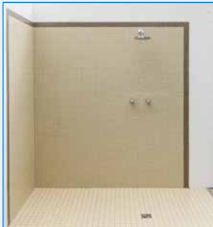
Bathroom completely tiled
