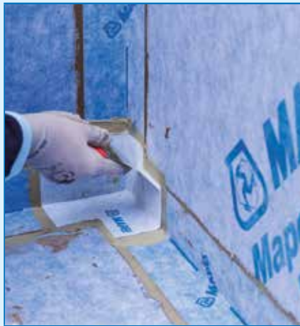
Application of MAPEGUARD IC in the internal corner with MAPEGUARD WP ADHESIVE
