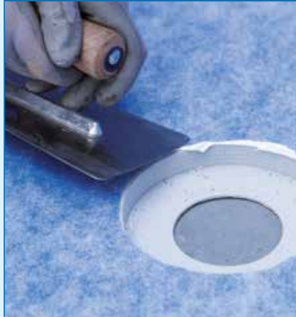
Press down MAPEGUARD WP 200 onto the drain
