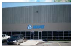
Calgary, Alberta Distribution Center
