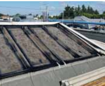
POSA BARRIERA VAPORE POLYVAP RADONSHIELD
