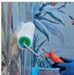
6 MAPECOAT DECOR PROTECTION felhordása Application of MAPECOAT DECOR PROTECTION
