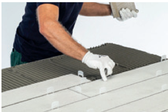
disposable clips installation
