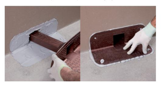
4. Spread a second coat of **Adesilex PG4** fresh on fresh to completely cover **Drain Front**.
