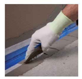
10. Apply a new layer of render on the parapet, or repair the old render removed before carrying out installation in the case of old structures.
