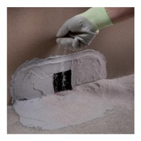
6. Once the reticulation process of **Adesilex PG4** has been completed, remove any loose quartz.
