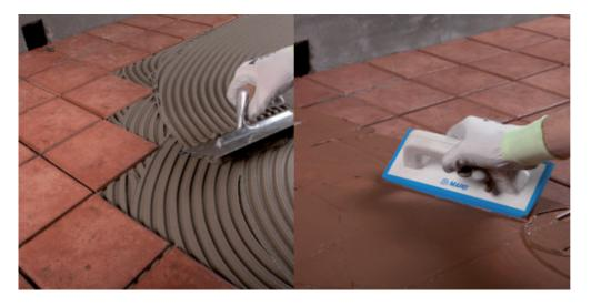
12. Bond the skirting boards and grout the vertical joints.
