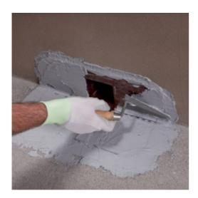
5. Smooth over with a flat trowel and, while the product is still fresh, sprinkle a layer of 0.5 spheroid quartz to form a rough layer to help the specified MAPEI waterproofing product form a good bond.
