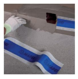
8. Lay **Mapeband** by pressing along the sides, making sure there are no creases or air bubbles.
