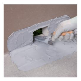
3. Place **Drain Front** in position and press down lightly so that it is embedded in **Adesilex PG4**.
