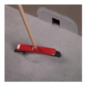
7. Apply the first coat of MAPEI waterproofing product on the clean, dry fillet between the horizontal and vertical surfaces
