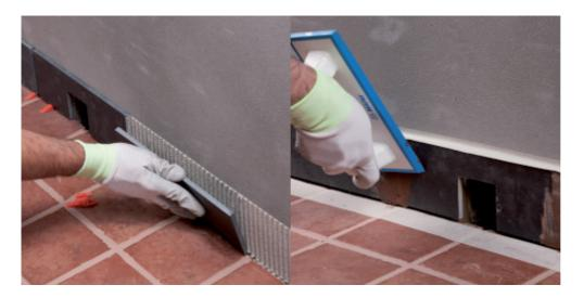
13. Seal with Mapesil AC or Mapesil AC Eco in correspondence with the skirting board-wall fillet joint.
