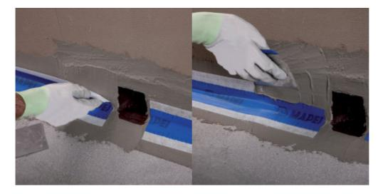
9. Spread a second layer of the specified MAPEI waterproofing product to completely cover the edges of the tape so they are sandwiched between the two layers of the cementitious mortar.
