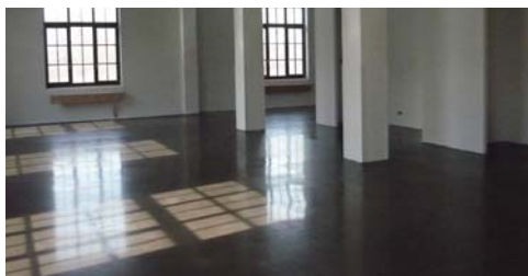
Antracit ULTRATOP MAPEFLOOR FINISH 50-nel kezelve.
