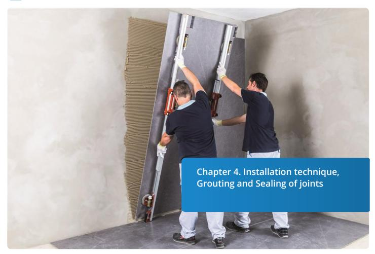
After selecting the adhesive (described in Chapter 2), the first step is to spread the adhesive on the substrate by using a spread with sloping notches (with a pitch of at least 10mm) to get better distribution of the adhesive.
