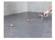
To make this operation easier, a special positioning tool may be used to correct the width of the grout line between adjacent tiles and bring the tiles to the position required.
