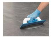
Clean the grouting by using a small amount of water and an abrasive pad (such as Scotch Brite®) followed by a firm cellulose sponge, taking care not to remove the grout.
