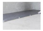
It is important to place the spacers in position before installing the tile. Ensure that the spacers are embedded in the adhesive.
