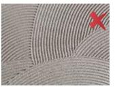
The adhesive must be spread in the same direction on the back of the tile and on the substrate (in straight lines parallel to the short side of the tile).
