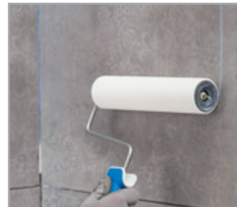
Application of MAPECOAT 4 LVT
