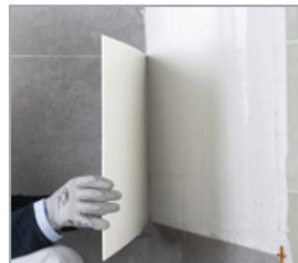
Installation of LVT/SPC with ULTRABOND ECO MS 4 LVT WALL
