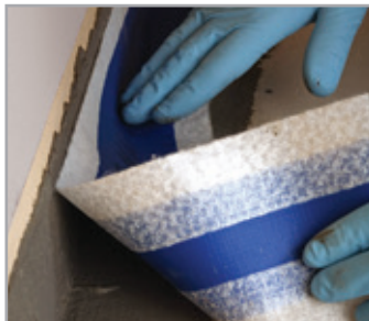
Application of MAPEBAND with MAPELASTIC SMART
