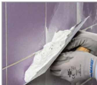
Wall and floor smoothing with PLANIPREP 4 LVT
