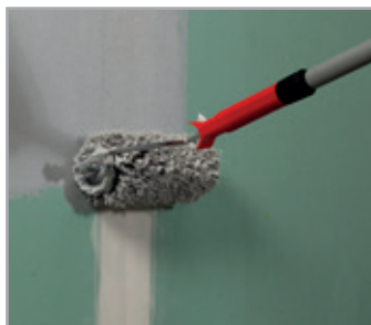
Spreading the first coat of MAPEGUM WPS
