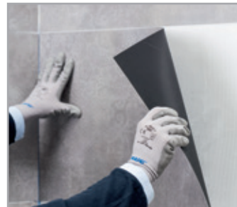
Installation of LVT with ULTRABOND ECO MS 4 LVT WALL
