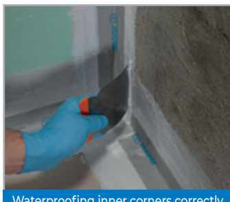
Waterproofing inner corners correctly by applying MAPEBAND PE120 and specially shaped pieces
