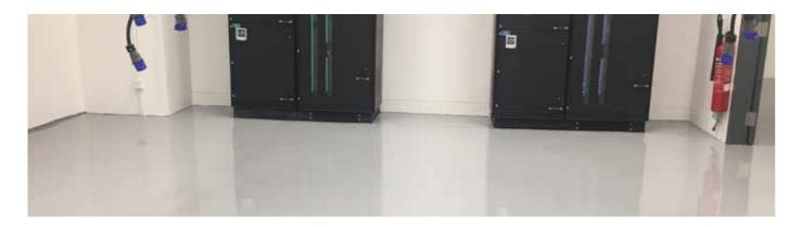
The semiconductor and electronics industry contain expensive equipment and components which are easily exposed to static charge within a given space and can be irreversibly damaged. In addition to damaged equipment, built-up charges can put workers and the facility at risk. Floor coatings with high performance ESD flooring are therefore a necessity.
