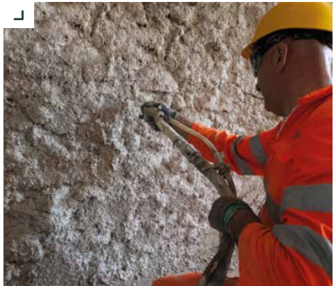
Application of PLANITOP INTONACO ARMATO by spray
