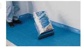
Go over the membrane with a float or roller and press it down (maximum 35 kg).
