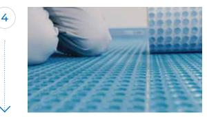
Apply **Mapeguard UM 35** rolls leaving a 3-5 mm gap between the sheets.
