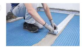
Waterproof joints between adjacent sheets with **Mapeband Easy**, bonded with **Mapeguard WP Adhesive** (3 mm notches trowel).
