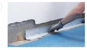
Perimetrally waterproof with **Mapeband Easy**, bonded with **Mapeguard WP Adhesive** (3 mm notches trowel).
