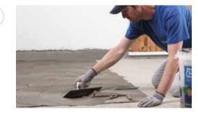
Spread the adhesive over the surface of the substrate with a 5 mm notches trowel.
