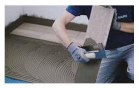
Install ceramic or stone tiles with a suitable **Mapei** adhesive of at least C2 class.
