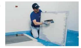
Install ceramic or stone tiles with a **Mapei** suitable adhesive of at least C2 class.
