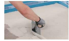
Spread the adhesive over the surface of the substrate with a 5 notches trowel.
