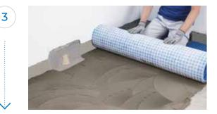
Lay **Mapeguard UM 35** membrane over the adhesive while it is still wet.
