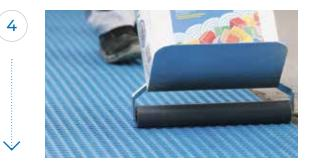
Go over the membrane with a float or roller and press it down (maximum 35 kg).
