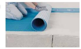
Lay **Mapeguard UM 35** membrane over the adhesive while it is still wet.
