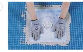
Waterproof drains with **Drain Vertical/Drain** Lateral.
