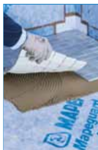
Installation of glass mosaic on Mapeguard WP 200
