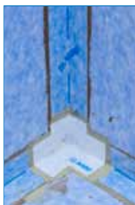
Detail of a waterproofed corner
