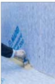
Application of Mapeguard WP Adhesive to bond Mapeguard ST
