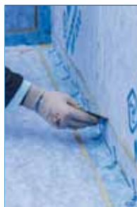
Application of Mapeguard ST
