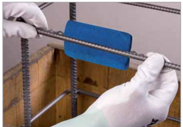
Application of Mapeshield I on a new structure
