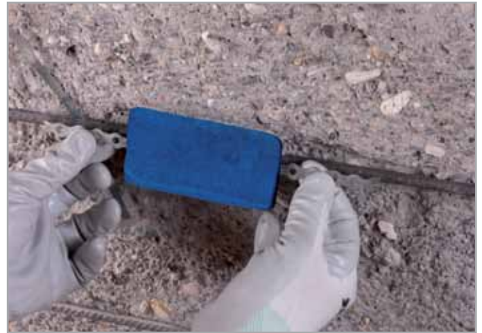
Application of Mapeshield I on a structure under repair
