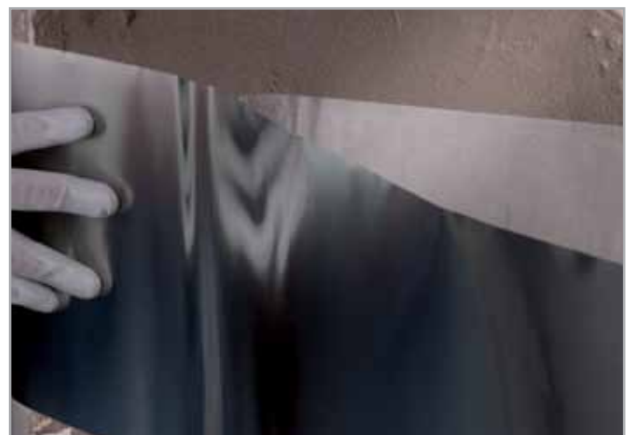
Application of Mapeshield E 25 on the external surface of the structure
