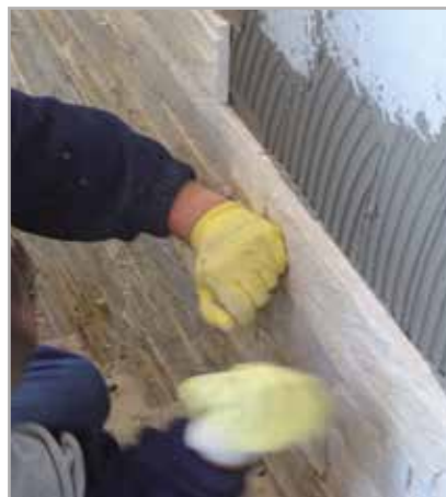
Fig. 7.10 Tapping a block of reconstituted stone into position
