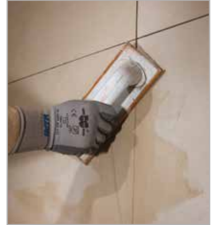
Fig. 6.4 - Grouting the joints with ULTRACOLOR PLUS
