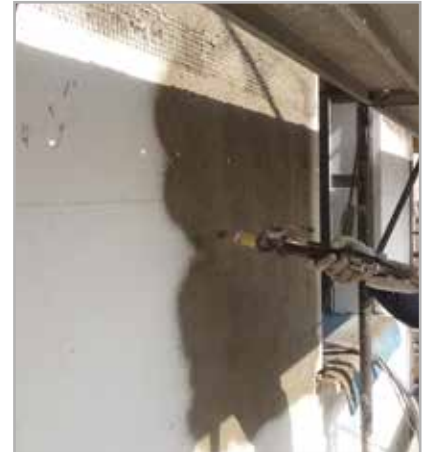
Fig. 5.7 - Application of PLANITOP HDM MAXI with a rendering machine
