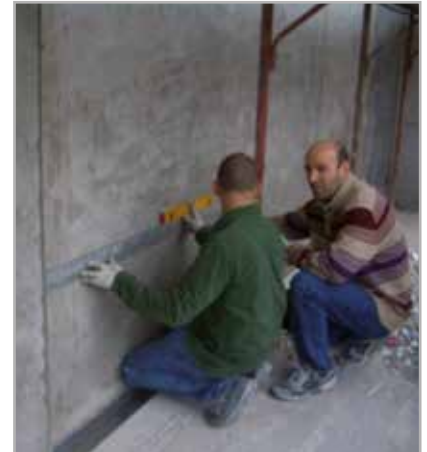
Fig. 5.1 - Checking the flatness of the substrate
