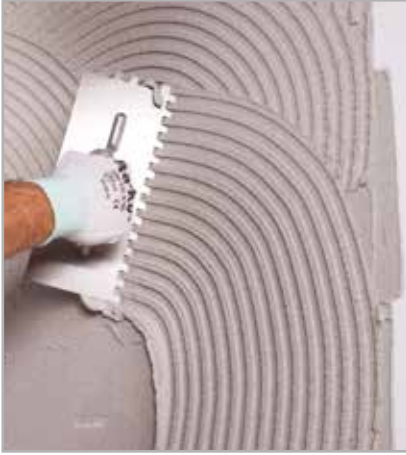
Fig. 5.4 - Spreading adhesive on the substrate
