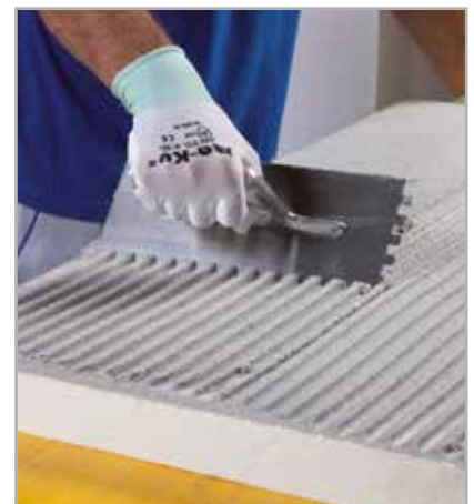
Fig. 5.3 - Spreading adhesive on the back of a panel
