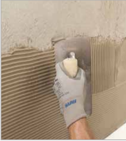
Fig. 6.2 - Application of ULTRALITE S2 on PLANITOP HDM MAXI structural render
