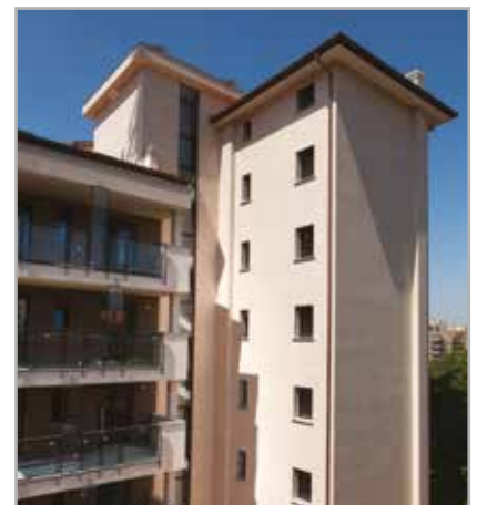
Fig. 1.3 - Residential building with MAPETHERM TILE SYSTEM
