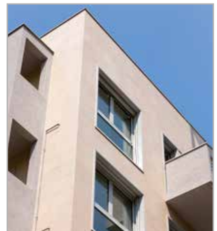
Fig. 3.3 - Residential building with MAPETHERM TILE SYSTEM
