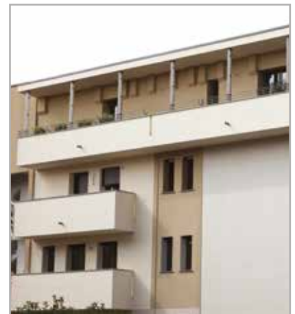
Fig. 1.2 - Residential building with MAPETHERM TILE SYSTEM
