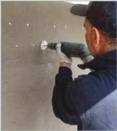
Fig. 5.11 - Application of MAPETHERM TILE FIX 15
