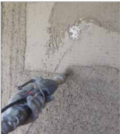
Fig. 5.12 - Application of the second layer of PLANITOP HDM MAXI
