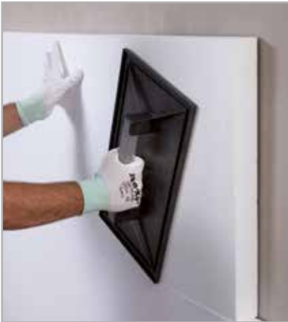
Fig. 5.5 - Installing a panel
