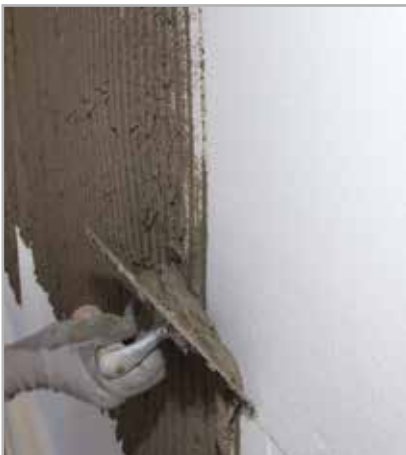
Fig. 5.6 - Application of PLANITOP HDM MAXI on the surface of EPS panels
