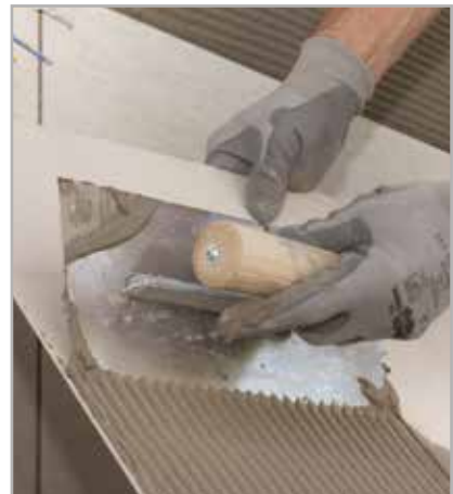
Fig. 5.14 - Application of ULTRALITE S2 on the back face of porcelain tiles
