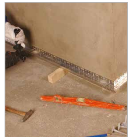
Fig. 4.16 - Positioning MAPETHERM BA support profiles
