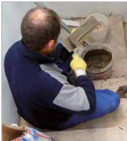
Fig. 7.7 Spreading adhesive on the back of the stone
