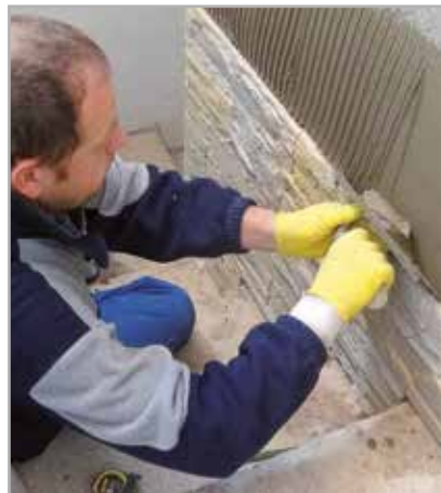
Fig. 7.8 Spreading adhesive on the substrate
