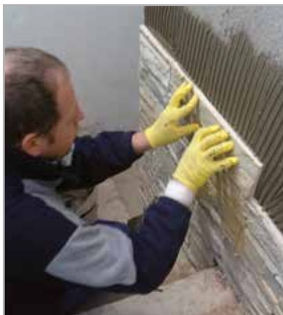
Fig. 7.9 Bonding stone using the double-buttering technique
