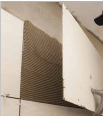
Fig. 6.3 - Installing porcelain tiles using the double-buttering method
