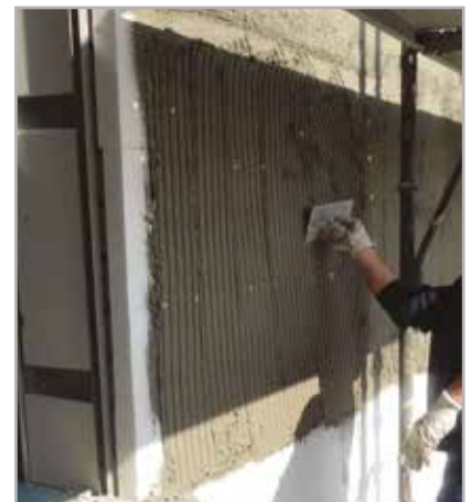
Fig. 5.8 - Spreading with a metal trowel
