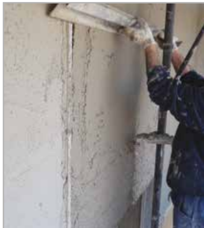
Fig. 5.13 - Levelling off the surface with a metal straight-edge
