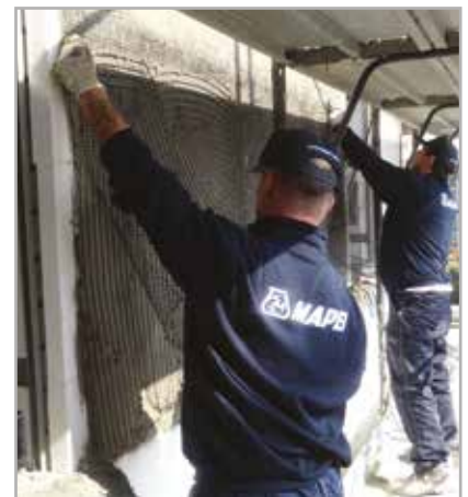
Fig. 5.9 - Positioning MAPEGRID G 120 reinforcing mesh
