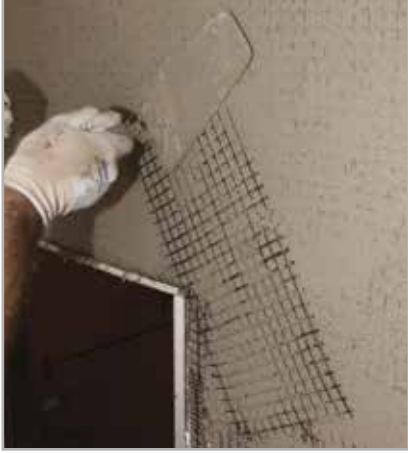
Fig. 5.10 - Positioning pieces of MAPEGRID G 120 around the edges of openings
