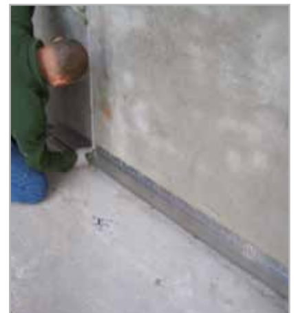
Fig. 5.2 - Applying a MAPETHERM BA support profile
