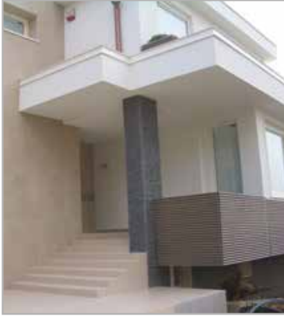
Fig. 3.1 - Residential building with MAPETHERM TILE SYSTEM
