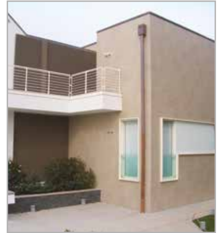
Fig. 1.1 - Residential building with MAPETHERM TILE SYSTEM
