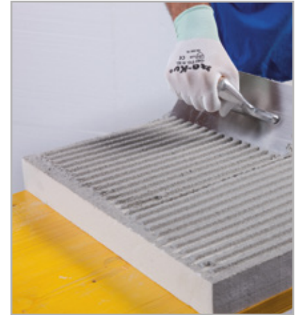
Fig. 6.5 - Adhesive spread evenly on the back of an insulating panel
