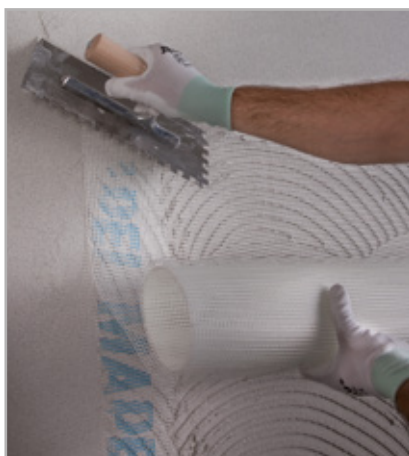
Fig. 6.13 - The edges of the mesh must overlap by at least 10 cm
