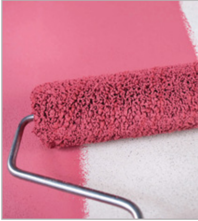
Fig 6.14 - Application of coloured primer
