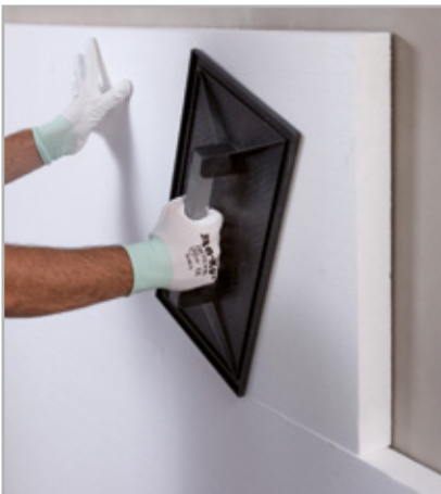
Fig. 6.8 - Pressing down the panel with a float
