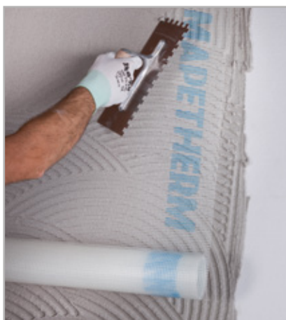
Fig. 6.12 - Application of MAPETHERM NET
