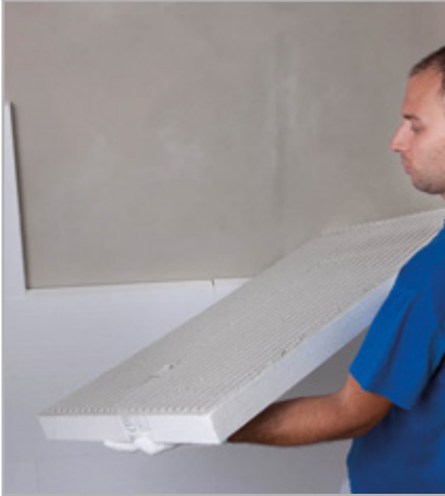
Fig. 6.7 - Panels bonded in place with staggered joints
