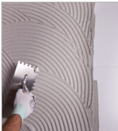
Fig. 6.11 - Application of the first coat of skimming compound
