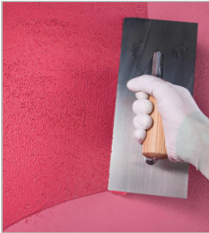
Fig 6.15 - Application of finishing render
