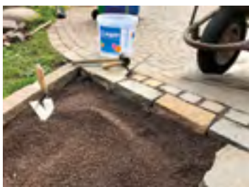
Prepare and apply the mix made up of 3/6 mm coarse stone chippings and Mapestone Joint
