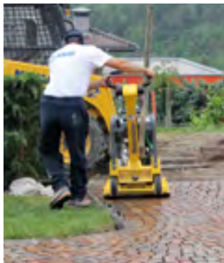
After wetting the surface, use a vibrating plate compactor
