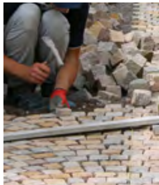
Install the stone blocks on a bed of 4/8 mm or 3/6 mm coarse stone chippings
