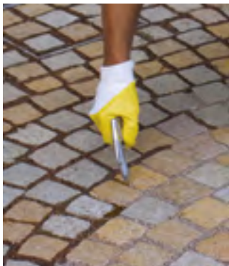
Fill the grout lines with Mapestone Joint
