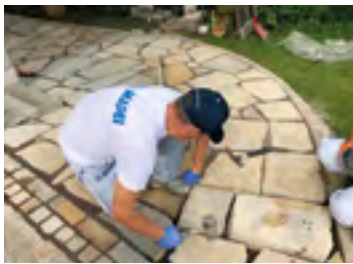
Install and tap down the slabs
