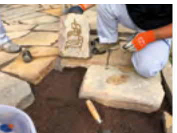
Apply Mapestone Joint on the back of the slabs
