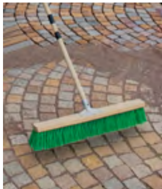
Fill the grout lines with 3/6 mm stone chippings
