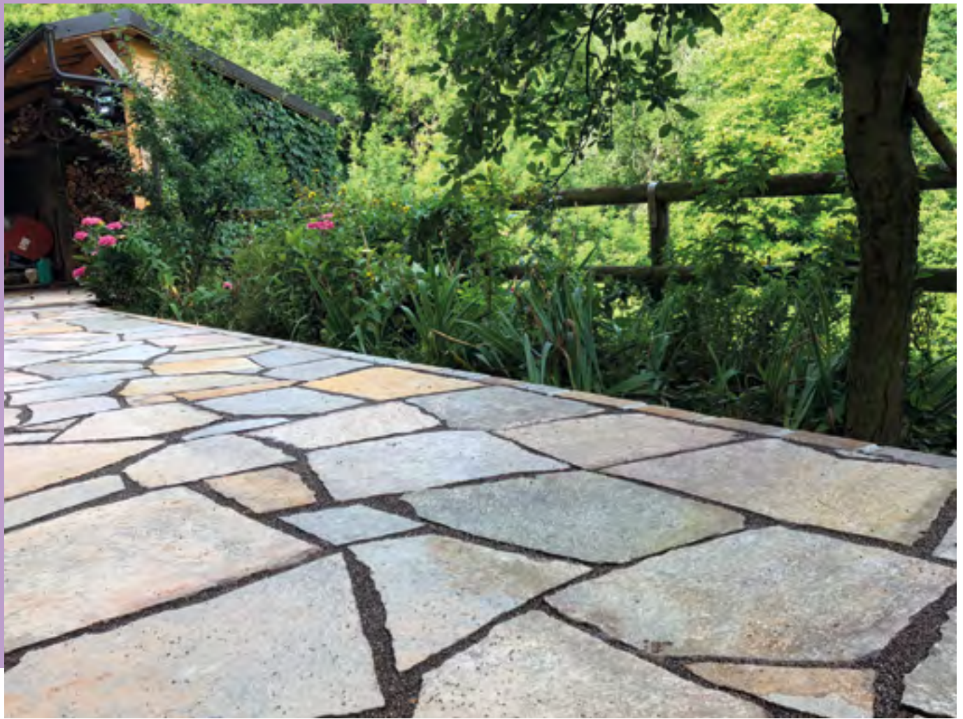
Fill the grouts with 3/6 mm coarse stone chippings and Mapestone Joint
