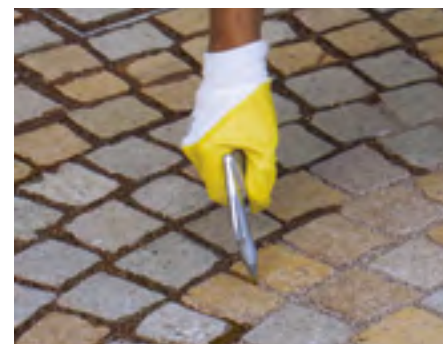
Fill the grouts with Mapestone Joint resin
