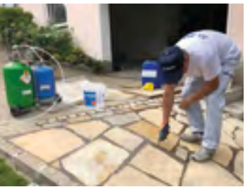
Fill the grouts with 3/6 mm coarse stone chippings and Mapestone Joint
