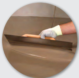
5. Spread the mixture using a notched trowel
