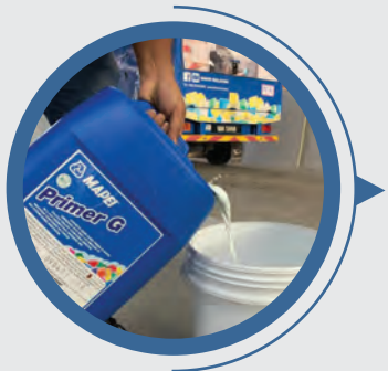
Dilute PRIMER G with water (1:1) and mix at low-speed until homogeneous.
