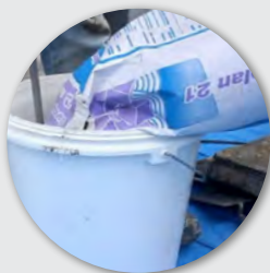
2. Gradually add one bag of Novoplan 21 while mixing continuously
