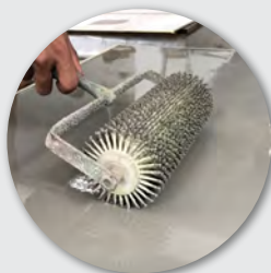
6. Spike roll to release entrapped air
