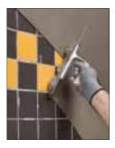
Water-repellent cementitious skimming mortar with a medium-textured natural finish for concrete, plastic coatings, glass and porcelain.
