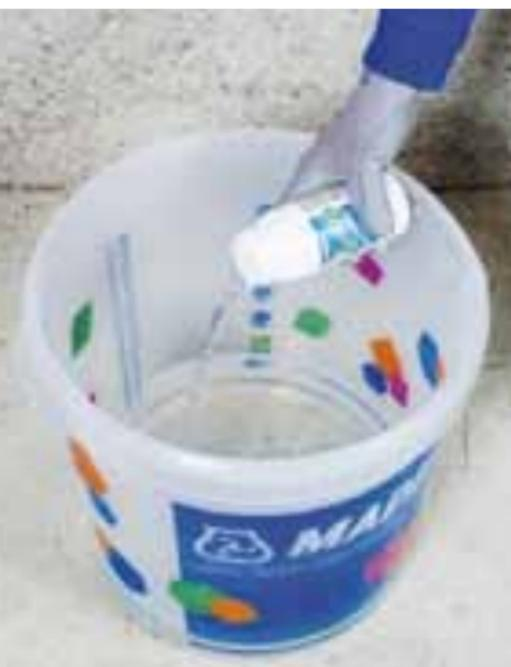
Adding **Mapetard ES** to the mixing water for **Planitop Smooth & Repair R4**
