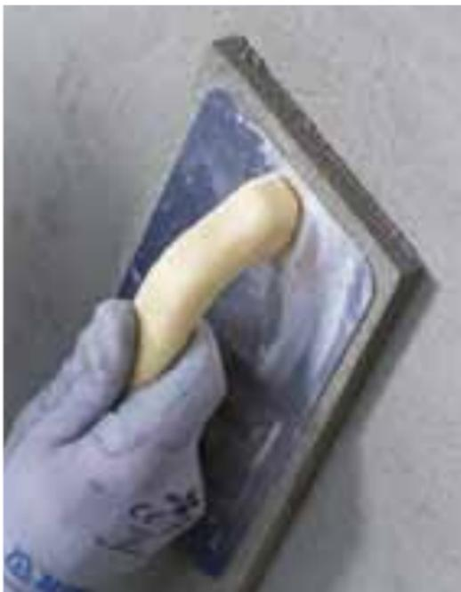
Floating the surface of **Planitop Smooth & Repair R4**
