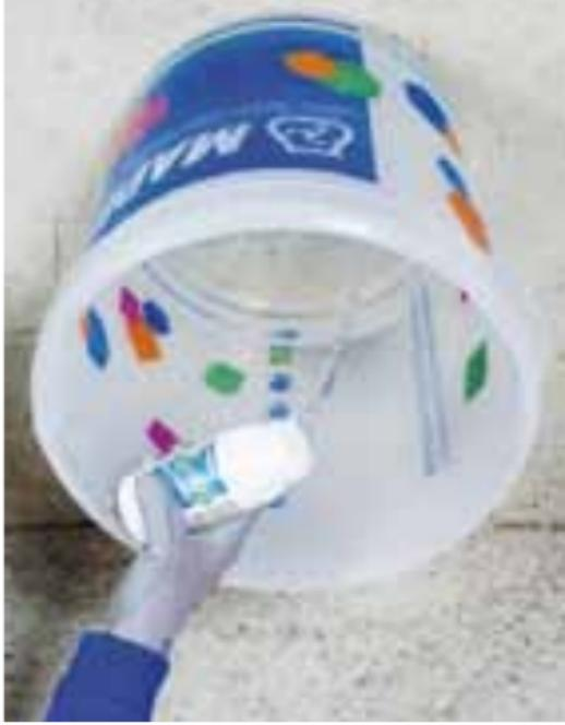
Adding **Plantop Smooth & Repair** to the mixing water admixed with **Mapetard ES**
