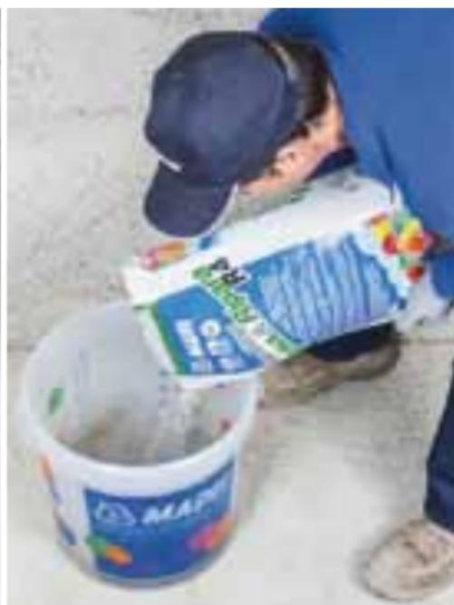
Adding **Planitop Smooth & Repair R4** to the mixing water admixed with **Mapetard ES**
