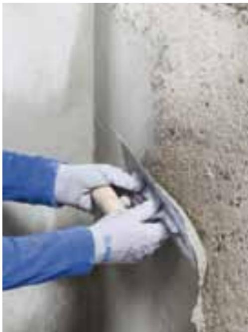
Application of **Planitop Smooth & Repair R4** with a finishing trowel
