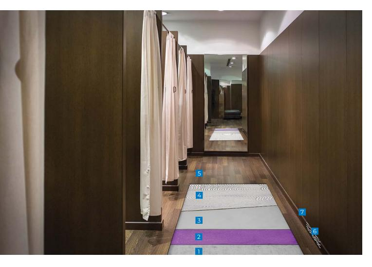
Heavy-traffic areas are where the majority of the traffic will be moving along a set path, time after time. The materials used to flatten and adhere these areas must be designed with a high compressive strength and stay where they are placed, even under heavy traffic conditions.
