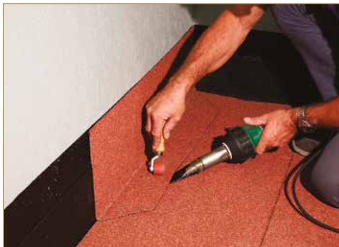
Figure 9.18: Welding the overlap on the flat surface
