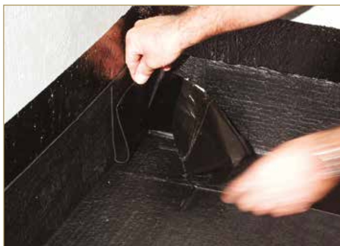
Figure 9.9: Removing the protective film
