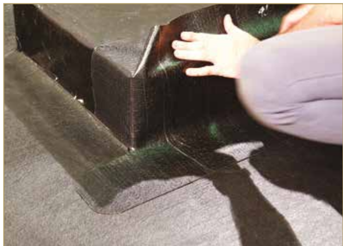
Figure 9.38: Folding the membrane on the upper edge
