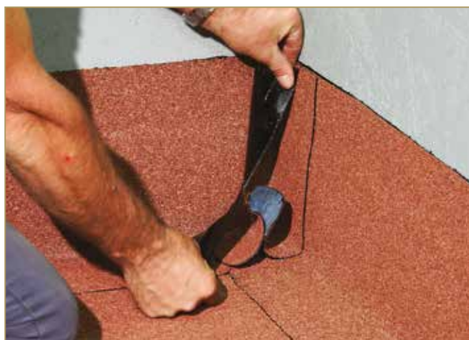
Figure 9.25: First gluing phase of the membrane patch
