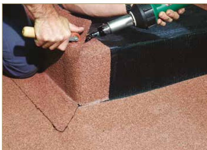
Figure 9.58: Hermetically closing and welding the corner
