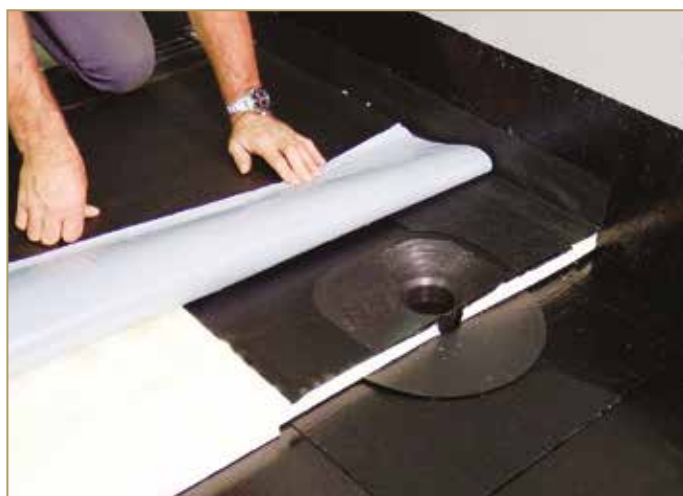
Figure 9.79: Positioning the first waterproof layer
