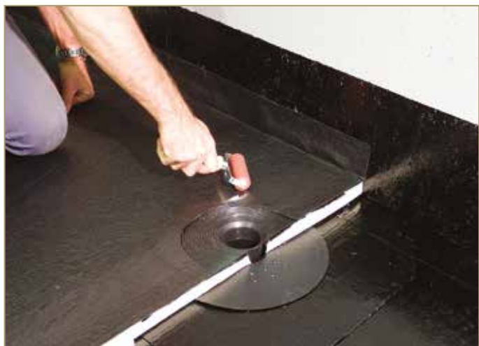
Figure 9.81: Membrane gluing and rolling
