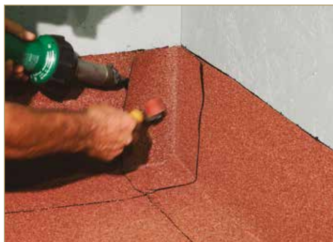
Figure 9.26: Welding the patch on the vertical wall
