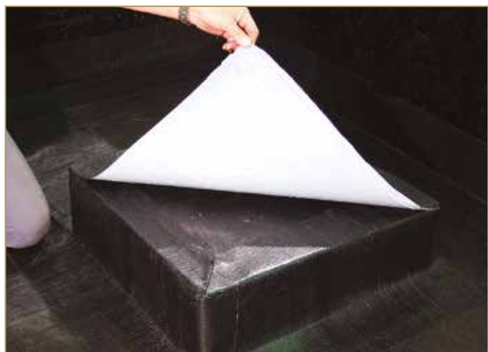
Figure 9.50: Preparing the top of the protruding structure
