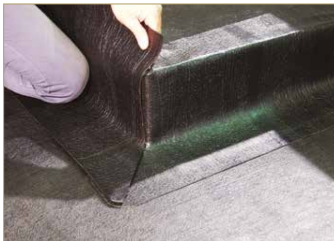
Figure 9.42: Gluing on the vertical wall of the up-turn
