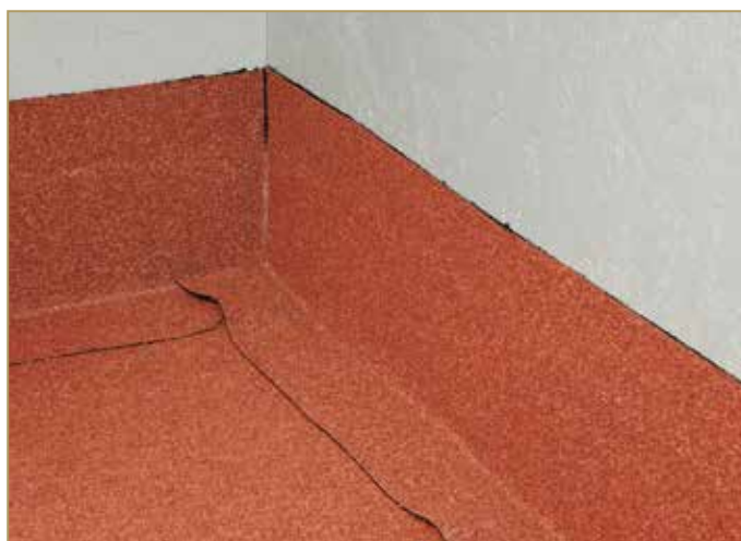
Figure 9.22: Vertical up-turn adhered to the wall
