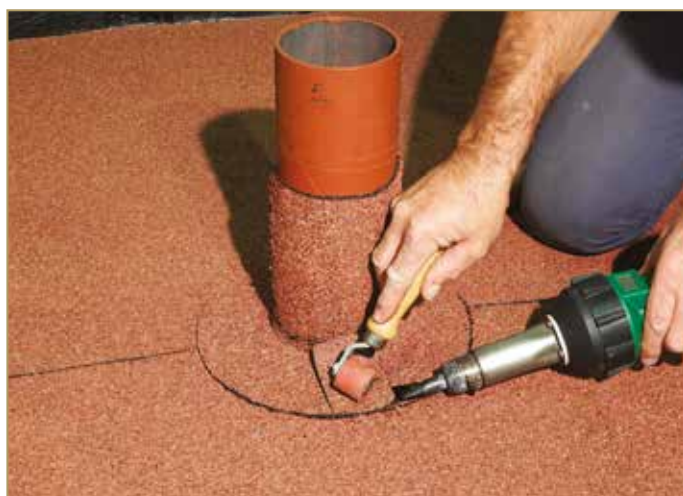
Figure 9.103: Closing weld of the patch cut
