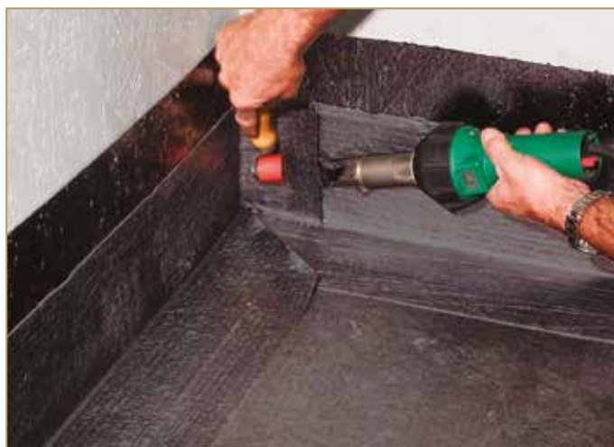
Figure 9.2: Up-turn vertical welding
