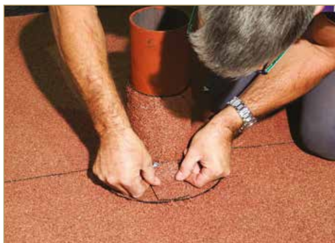
Figure 9.102: Positioning the closing patch
