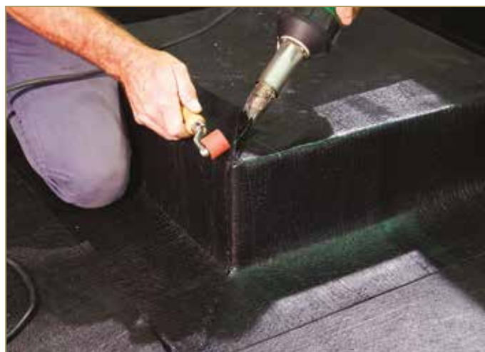
Figure 9.45: Welding the upper corner
