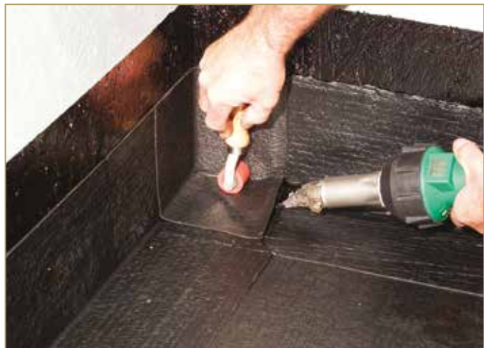
Figure 9.11: Hermetically closing and welding the corner
