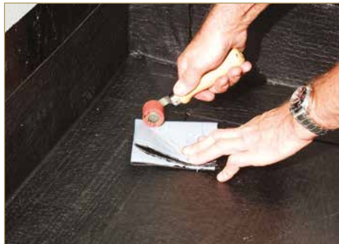
Figure 9.6: Rolling to mark the 4 corner portions
