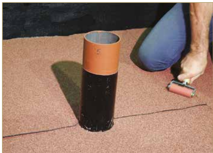
Figure 9.93: Rolling the overlaps
