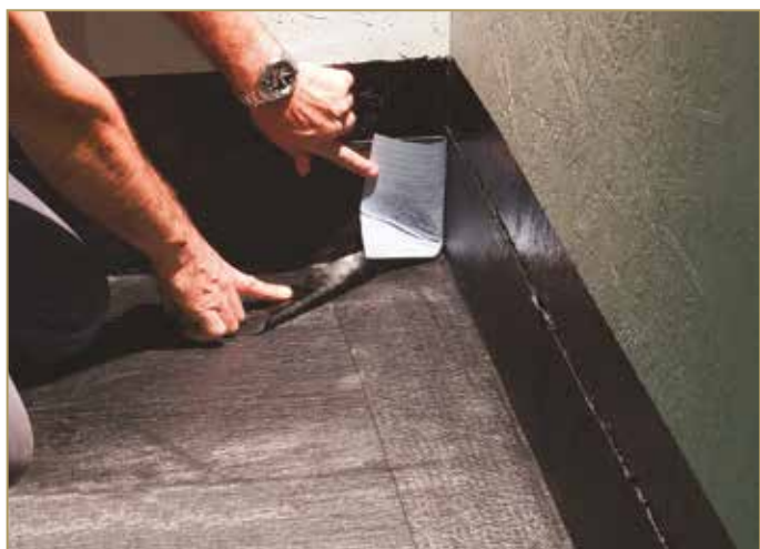
Figure 9.1: Preparation of the internal corner
