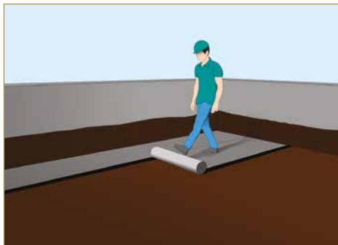
Figure 7.8: Unroll the membrane in its final position
