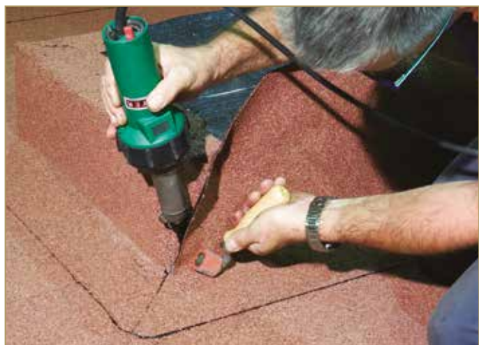
Figure 9.62: Welding the vertical overlap
