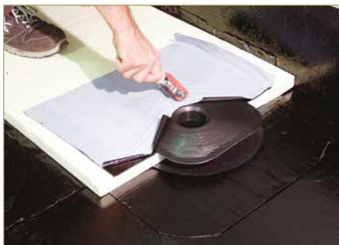
Figure 9.77: Replacing the protective film and rolling to glue outlet
