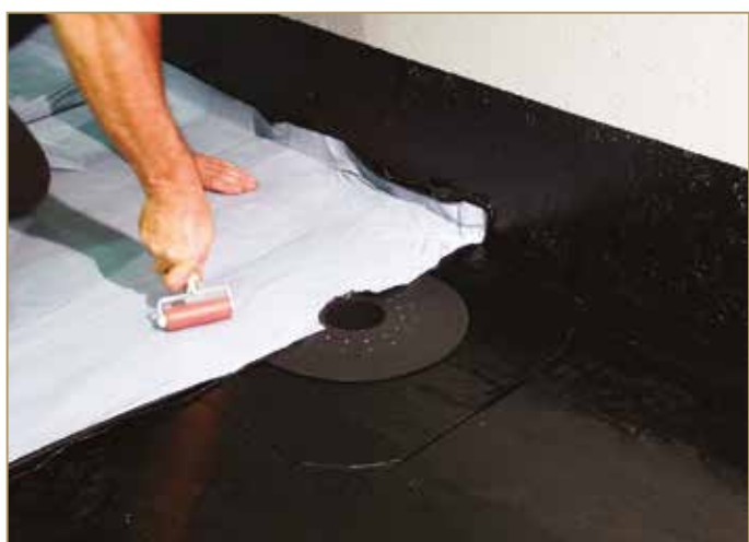
Figure 9.73: Positioning the ADESO vapour barrier and rolling
