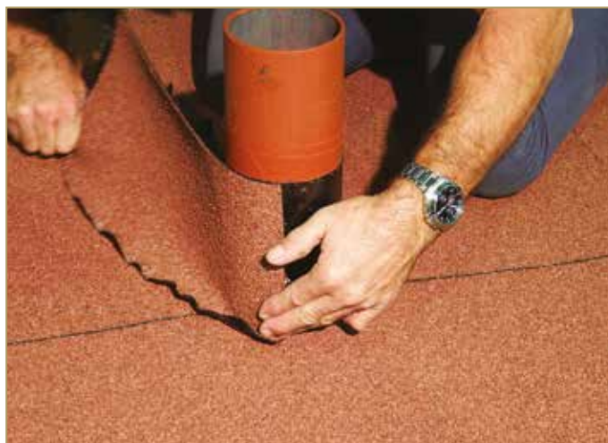
Figure 9.96: Gluing the vertical up-turn on the tube
