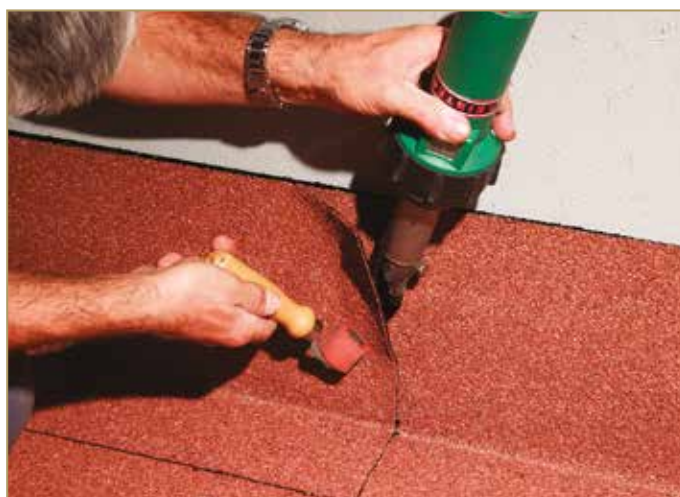
Figure 9.32: Up-turn at vertical welding
