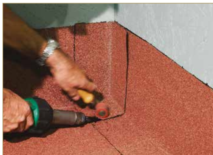
Figure 9.28: Hermetically closing and welding the corner
