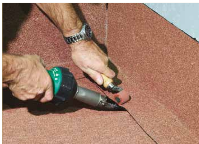
Figure 9.23: Welding the overlap on the flat surface
