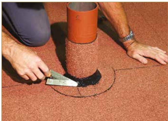
Figure 9.105: Levelling the POLYDETAIL MS
