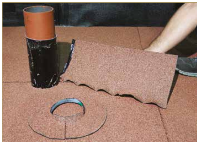
Figure 9.95: Preparing the elements to line the tube
