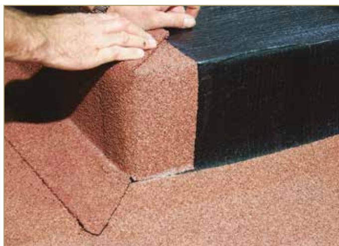
Figure 9.57: Folding the membrane on the upper edge
