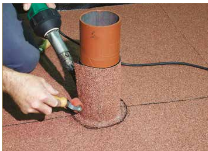
Figure 9.99: Welding the overlap on the vertical tube
