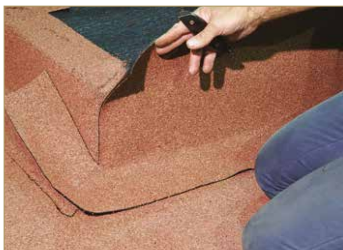
Figure 9.59: Preparing and gluing the adjacent vertical up-turn
