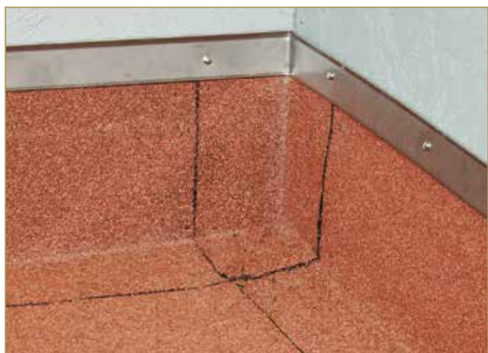
Figure 9.33: Fixing the termination profile to the wall
