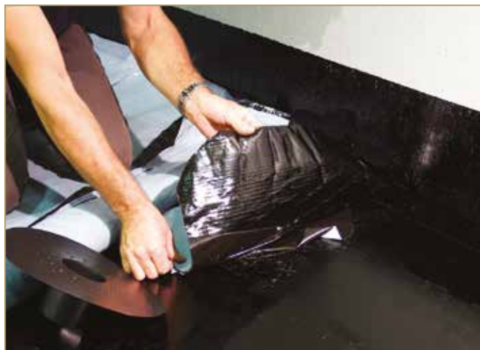
Figure 9.70: Positioning the membrane and removing the protective film
