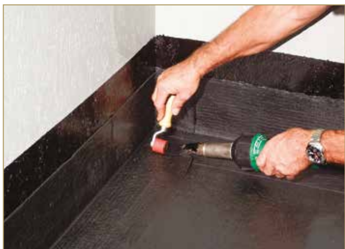
Figure 9.3: Flat welding
