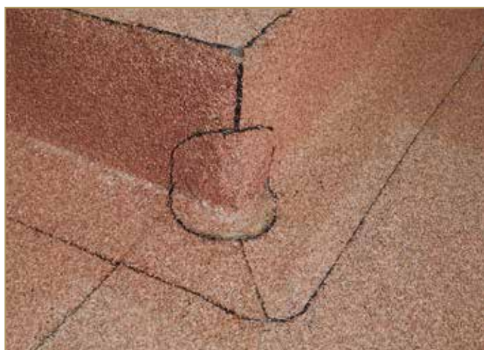
Figure 9.68: Finished external corners
