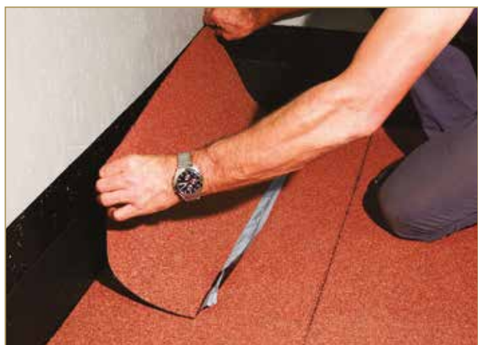
Figure 9.15: Positioning and gluing on the vertical up-turn
