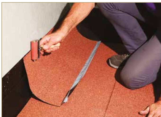
Figure 9.16: Rolling the top part
