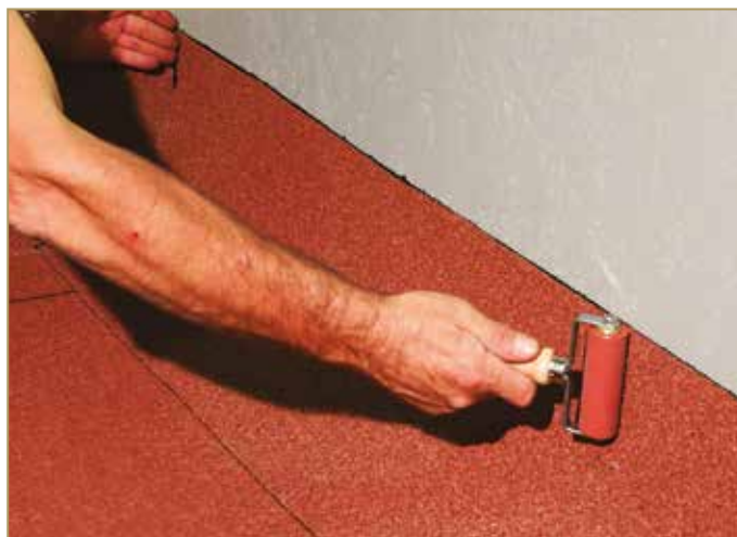
Figure 9.20: Rolling the vertical detail
