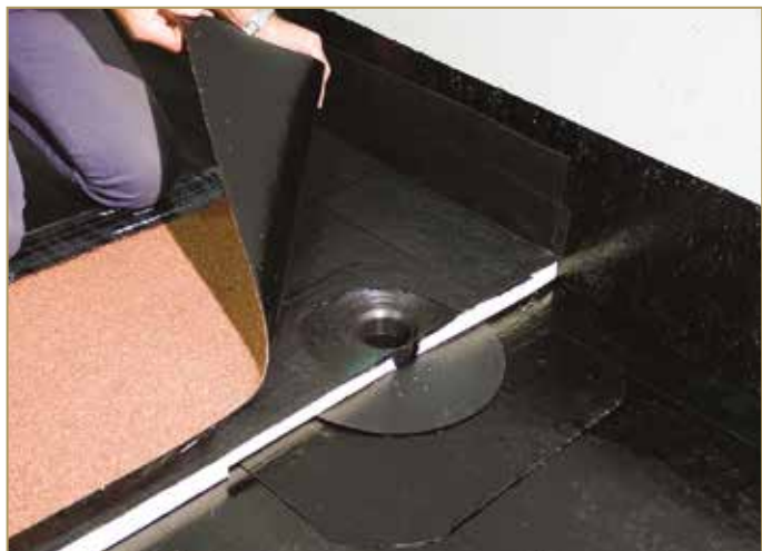
Figure 9.83: Laying the second waterproof layer with slate chipping finish
