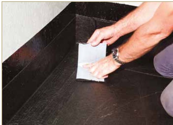
Figure 9.5: Folding the patch of membrane into 4 parts
