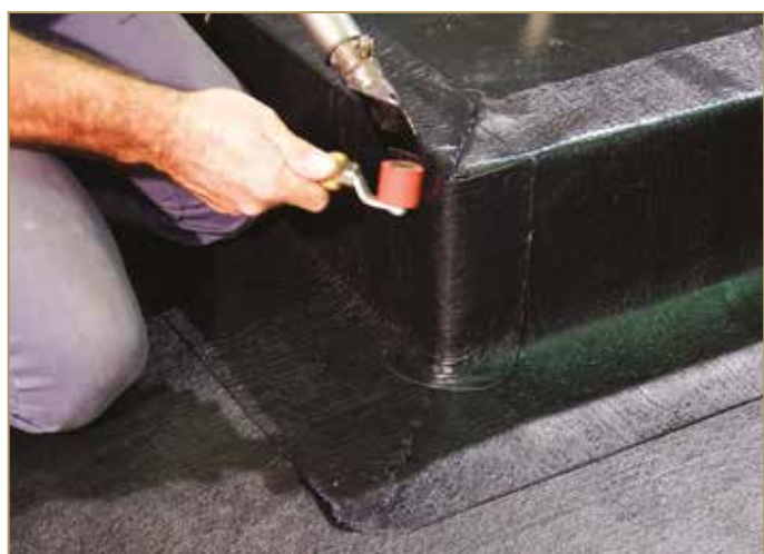
Figure 9.48: Welding the patch on the vertical wall
