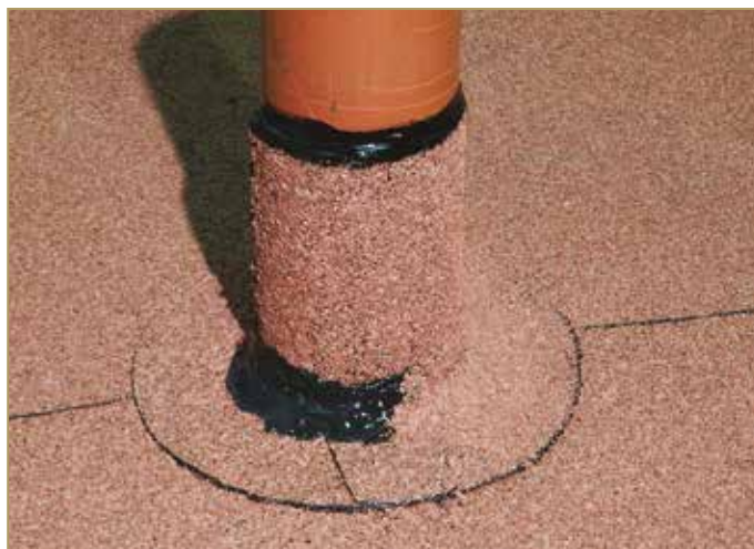
Figure 9.106: Top seal and aesthetic finish of the seal with slate chippings
