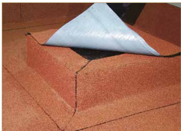
Figure 9.64: Preparing the base end closure
