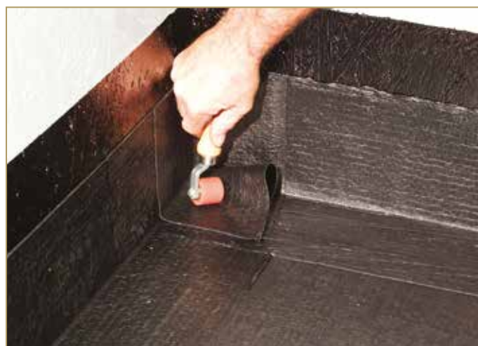
Figure 9.10: Horizontal gluing and rolling
