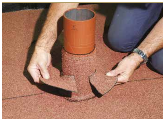
Figure 9.100: Positioning the covering patch
