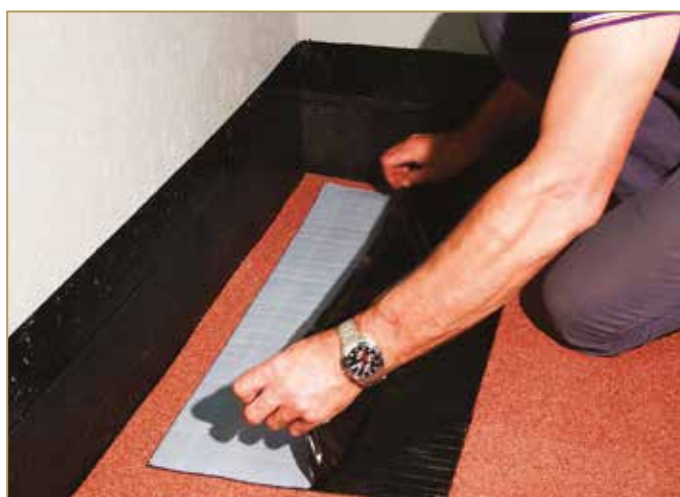
Figure 9.14: Partially removing the protective film
