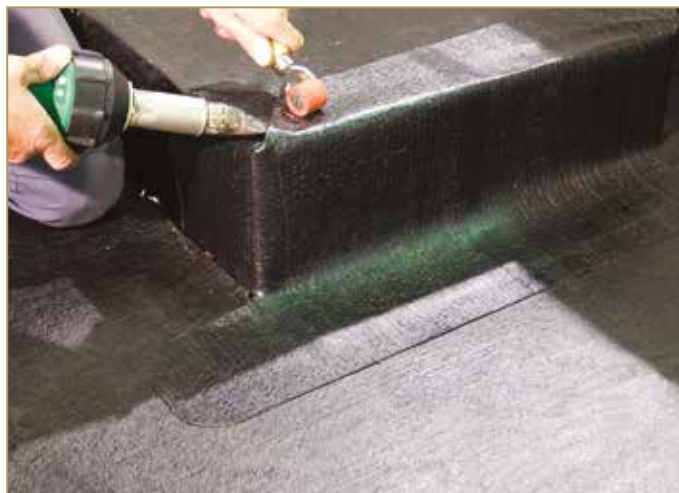
Figure 9.39: Hermetically closing and welding the upper corner
