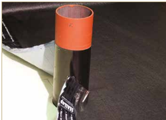
Figure 9.87: Positioning and cutting the first waterproof layer
