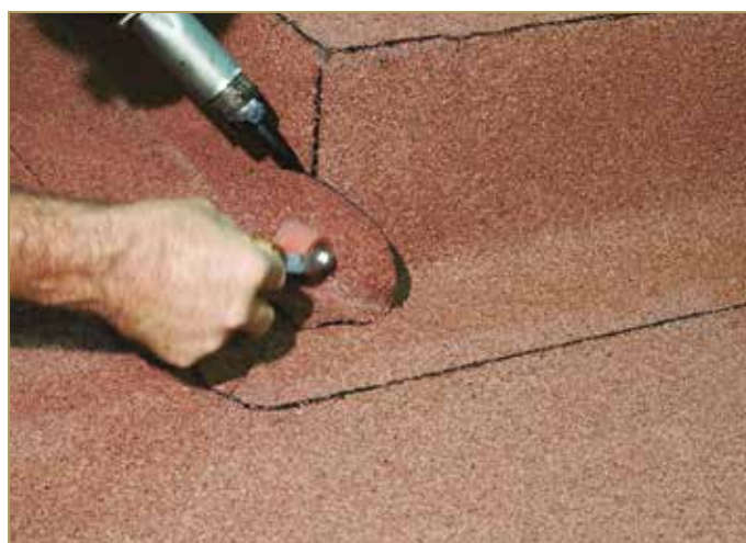
Figure 9.67: Welding the patch
