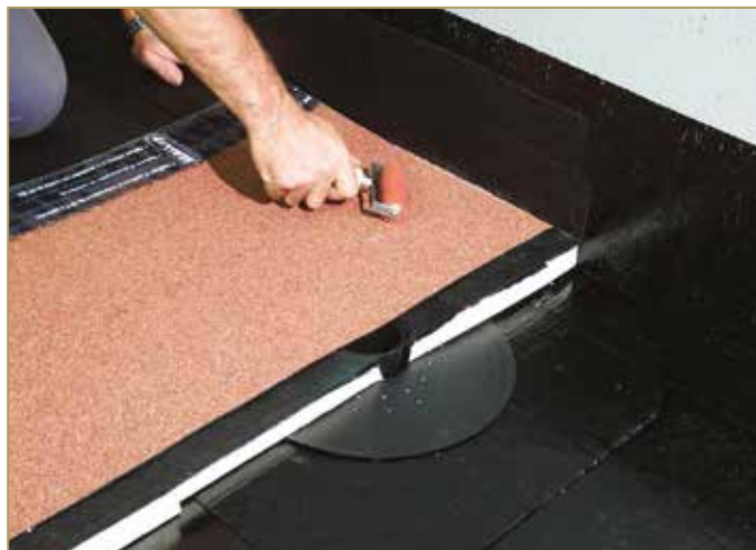
Figure 9.84: Rolling and gluing on the flat surface
