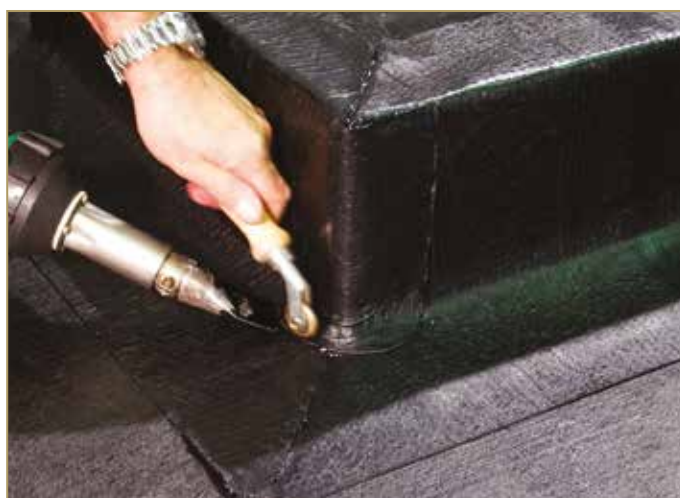
Figure 9.49: Welding the patch on the flat surface
