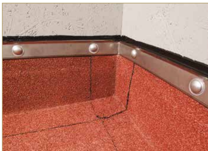
Figure 9.35: Completed internal corner with profile and studs
