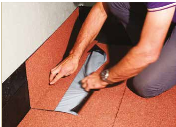
Figure 9.17: Removing the protective film
