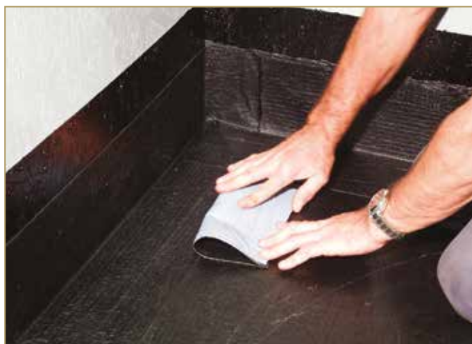
Figure 9.4: Cutting a 20x20 cm patch of membrane
