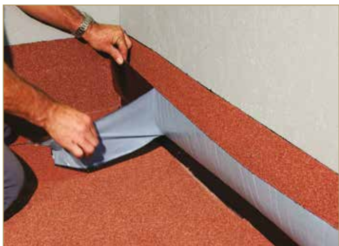
Figure 9.21: Total removal of the release film
