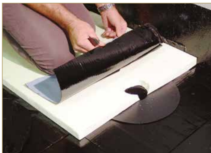
Figure 9.75: Positioning the membrane under the outlet
