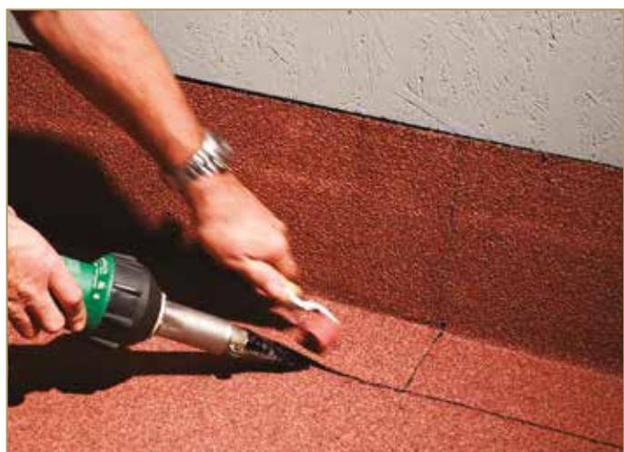
Figure 9.31: Welding the overlap on the flat surface
