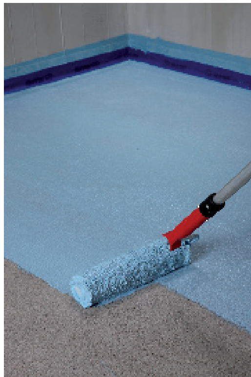
Application of the first coat of Mapelastc AquaDefense
