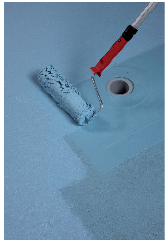
Application of the second coat of Mapelastc AquaDefense
