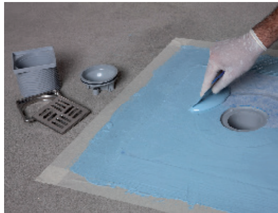
Impregnating Drain Vertical fabric with Mapelastc AquaDefense
