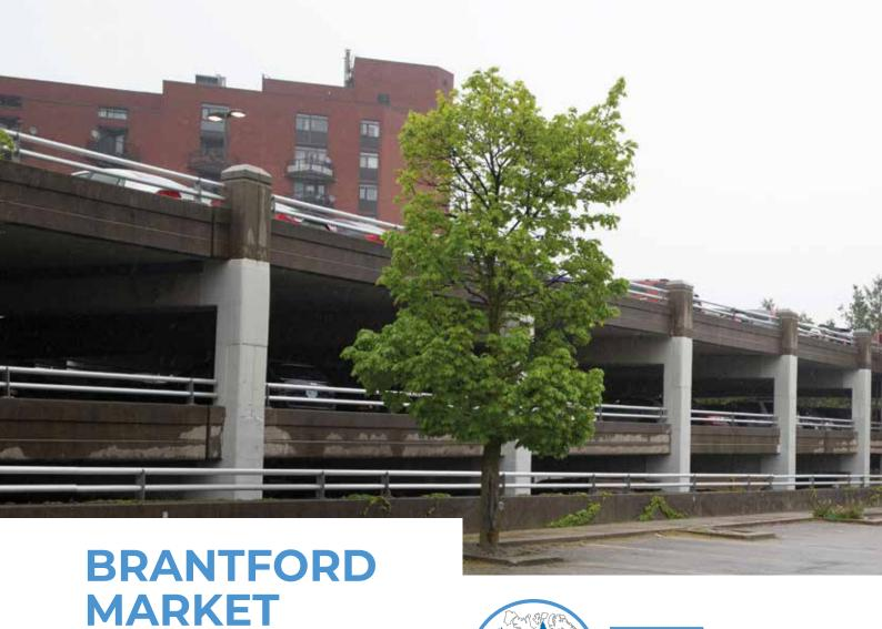
The concrete structure of the shopping centre's multi-storey carpark is made up of more than 200 columns and was upgraded and strengthened by applying products from the FRP System range of composites made from high-strength fibres and polymer resins.
